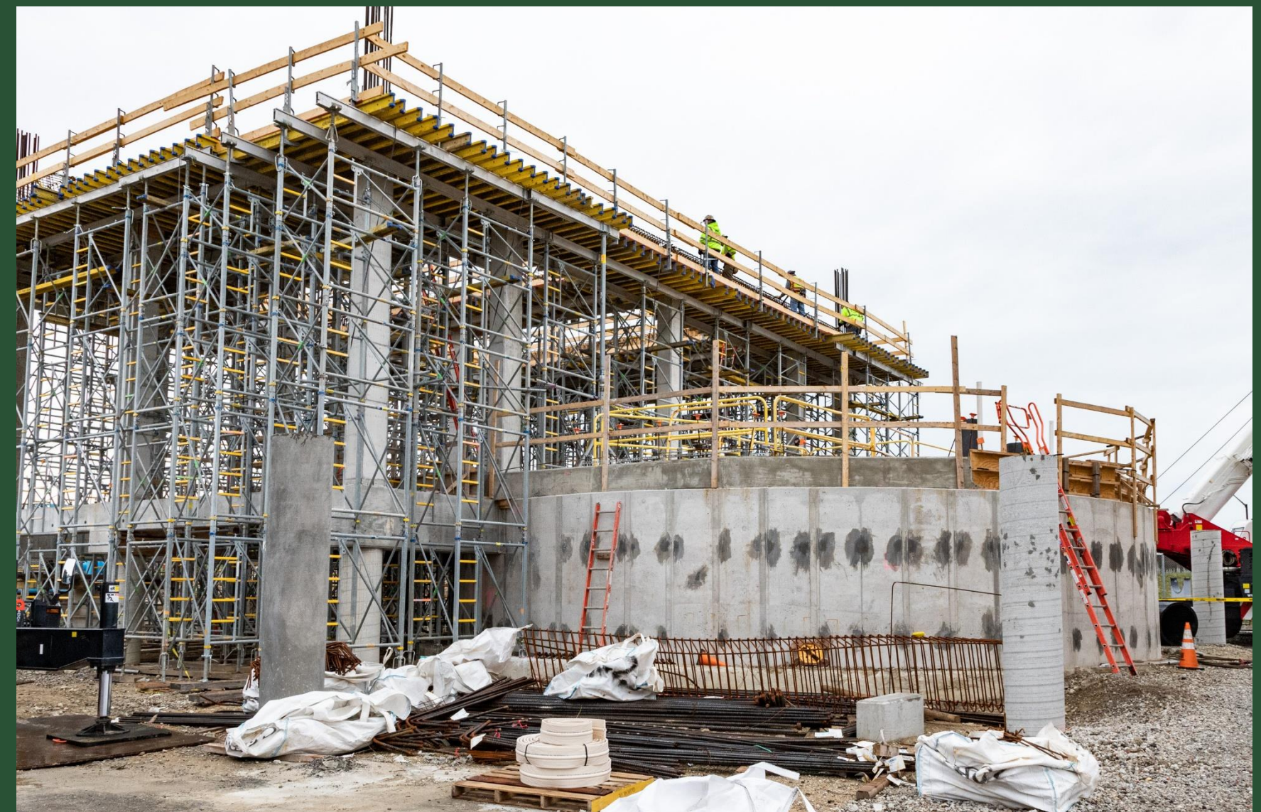
Pump Station Construction Near BP1 (March 2023)
