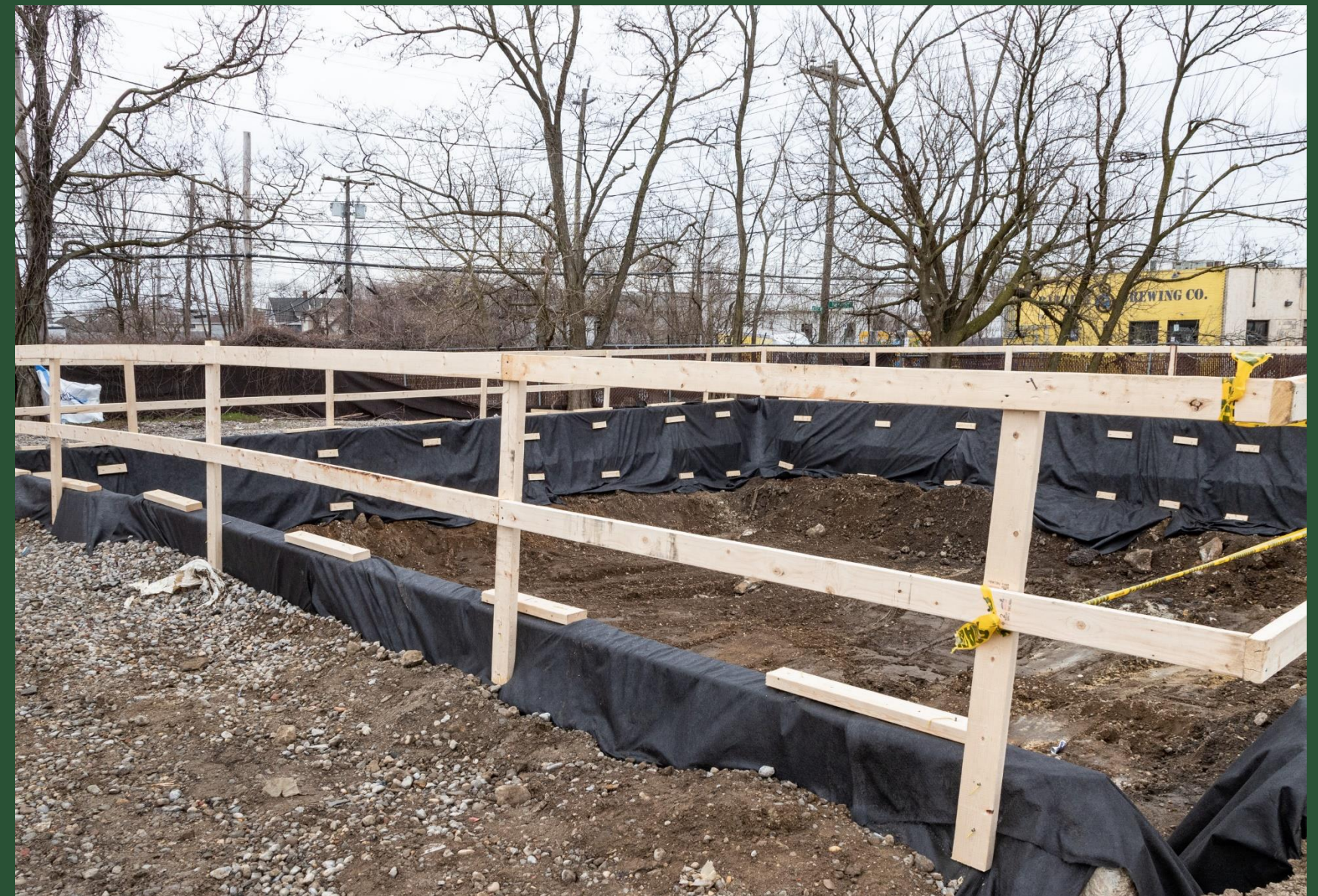
BP4 Construction Activities (March 2023)
