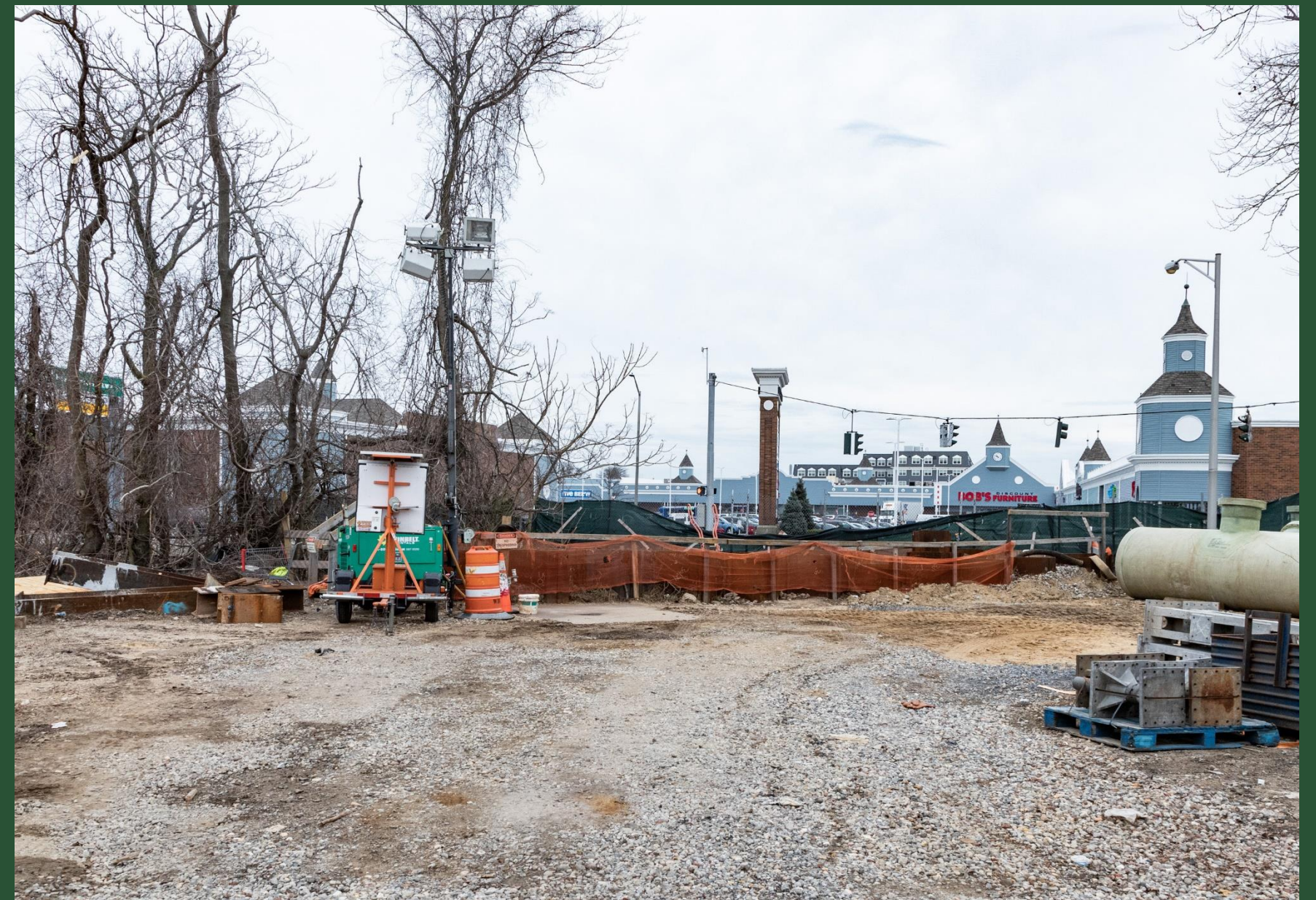
Pit O Construction Site (March 2023)
