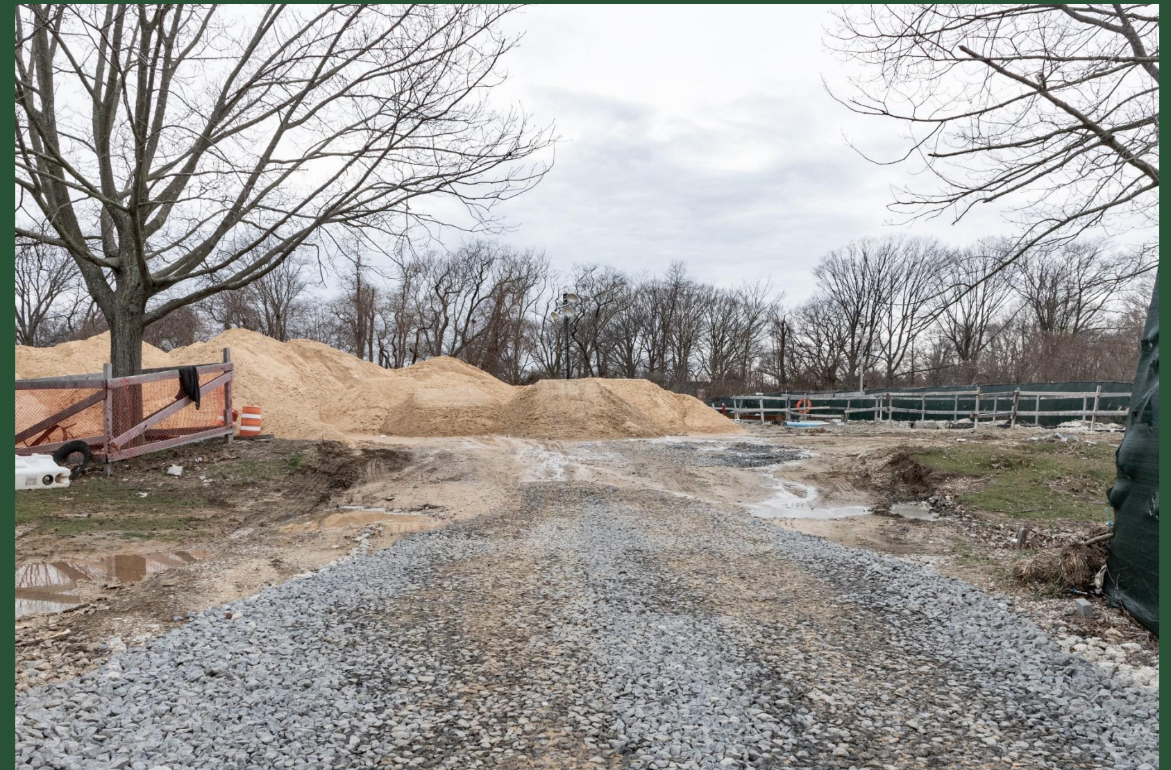
Construction Site at CC3 (February 2023)
