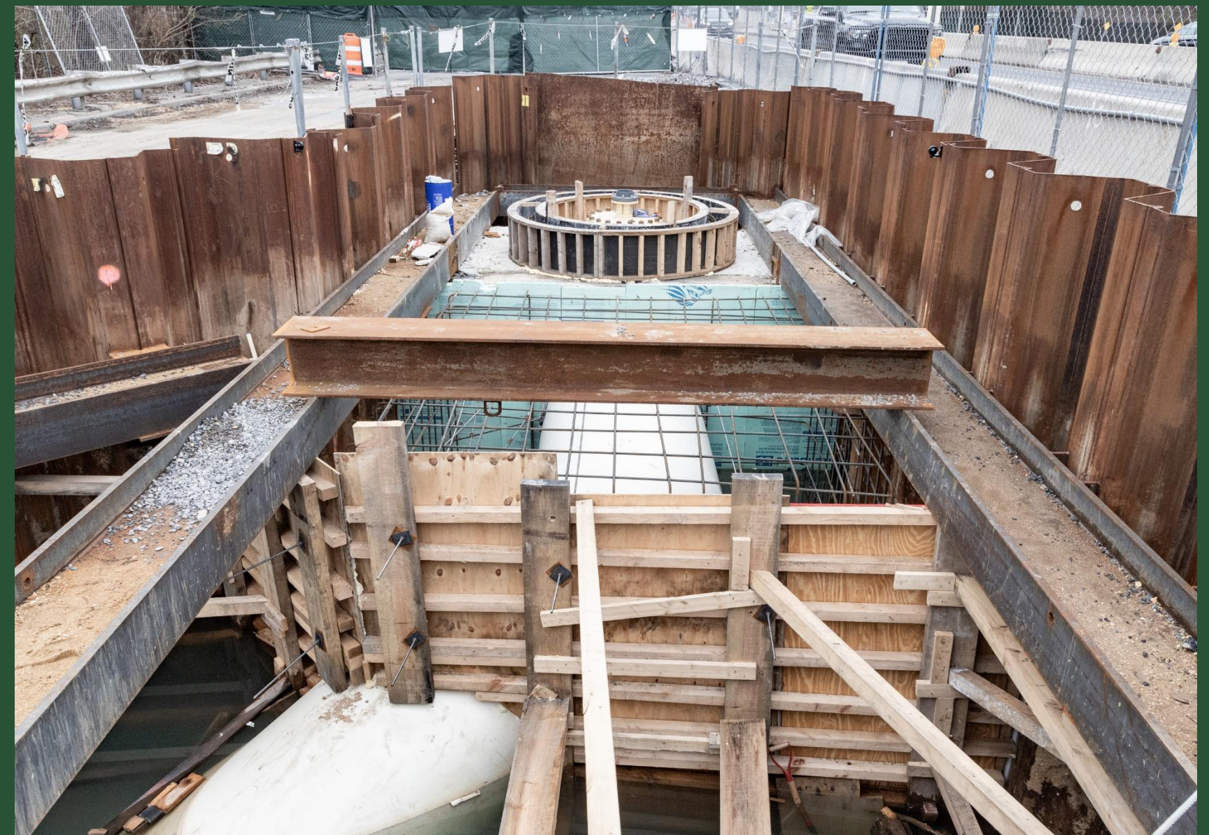
SOE at Pit W (March 2023)
