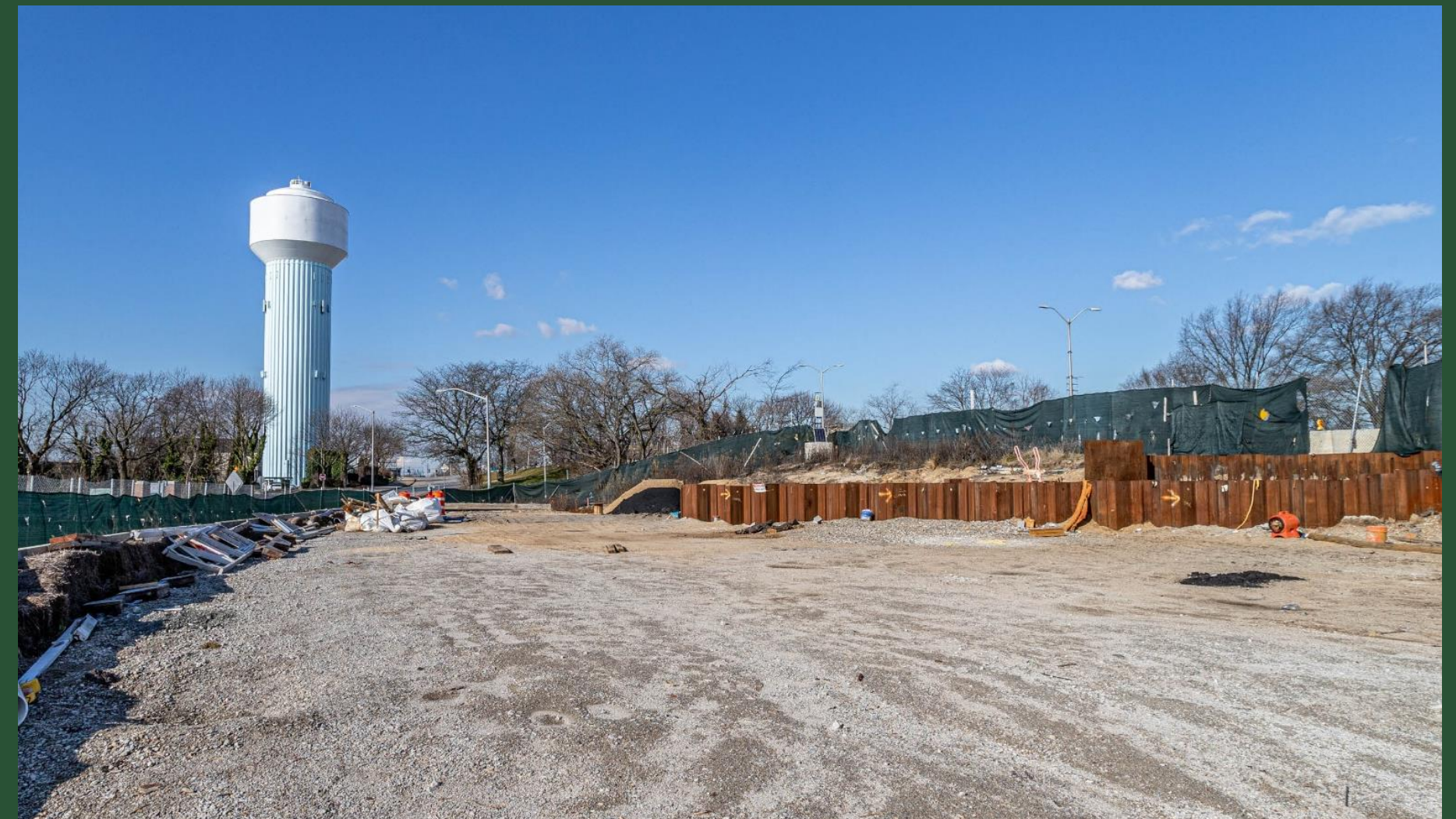
Construction Site at BP9 (January 2023)
