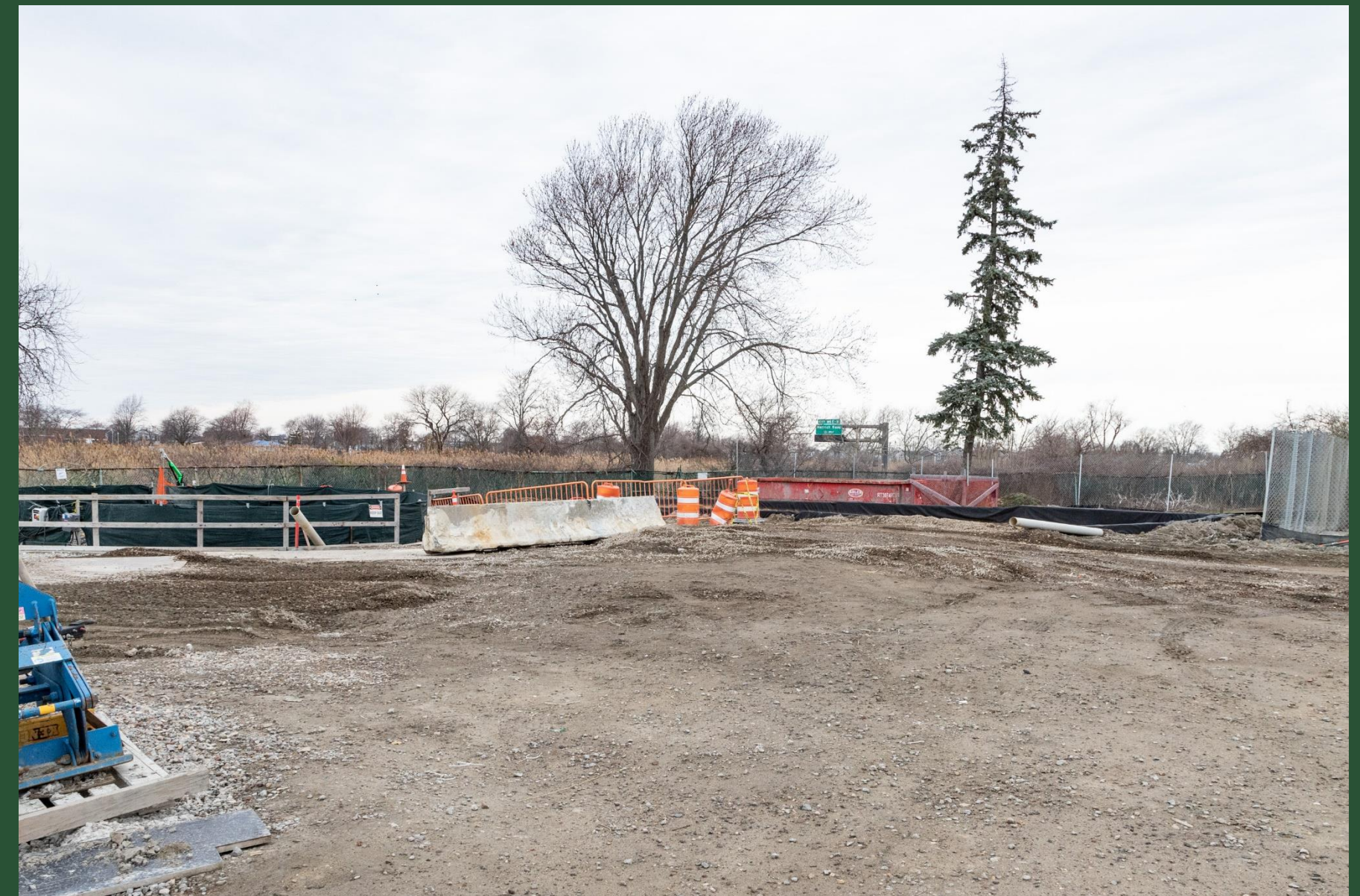
Construction Site at CC2 (March 2023)
