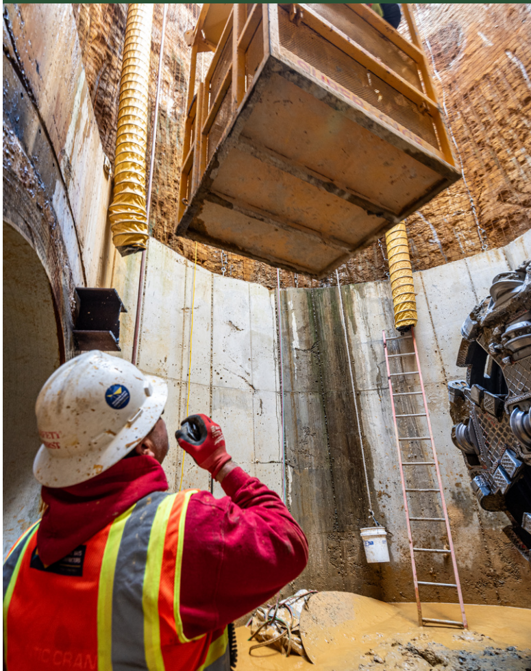
Inside the Shaft at Bay Park Shaft 7
