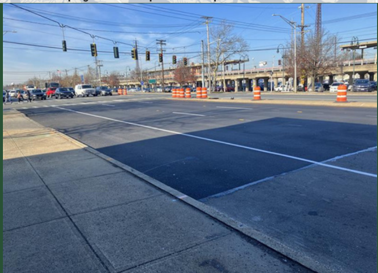
Final Roadway Restoration at Pit GG
