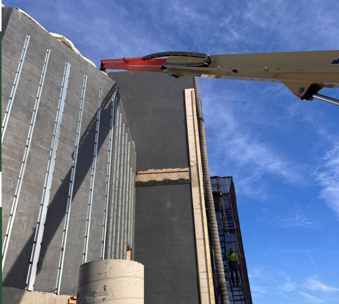
Exterior of the new Effluent Diversion Pump Station at SSWRF (November 2023)
