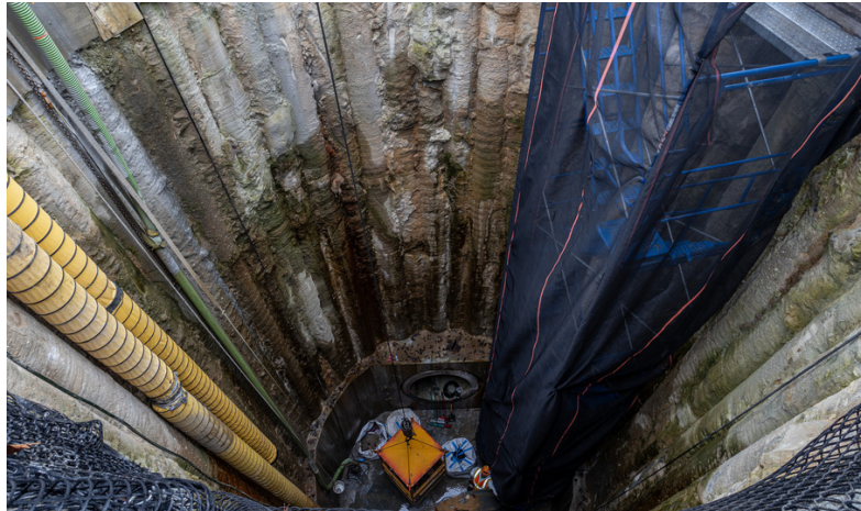
Cedar Creek Shaft 3 (December 2023)
