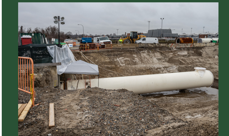
Pipe Installation Near CC1 (December 2024)
