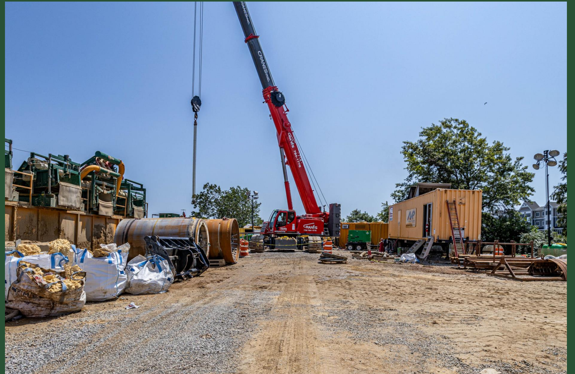
Post Microtunneling Activities at BP5 (July 2023)
