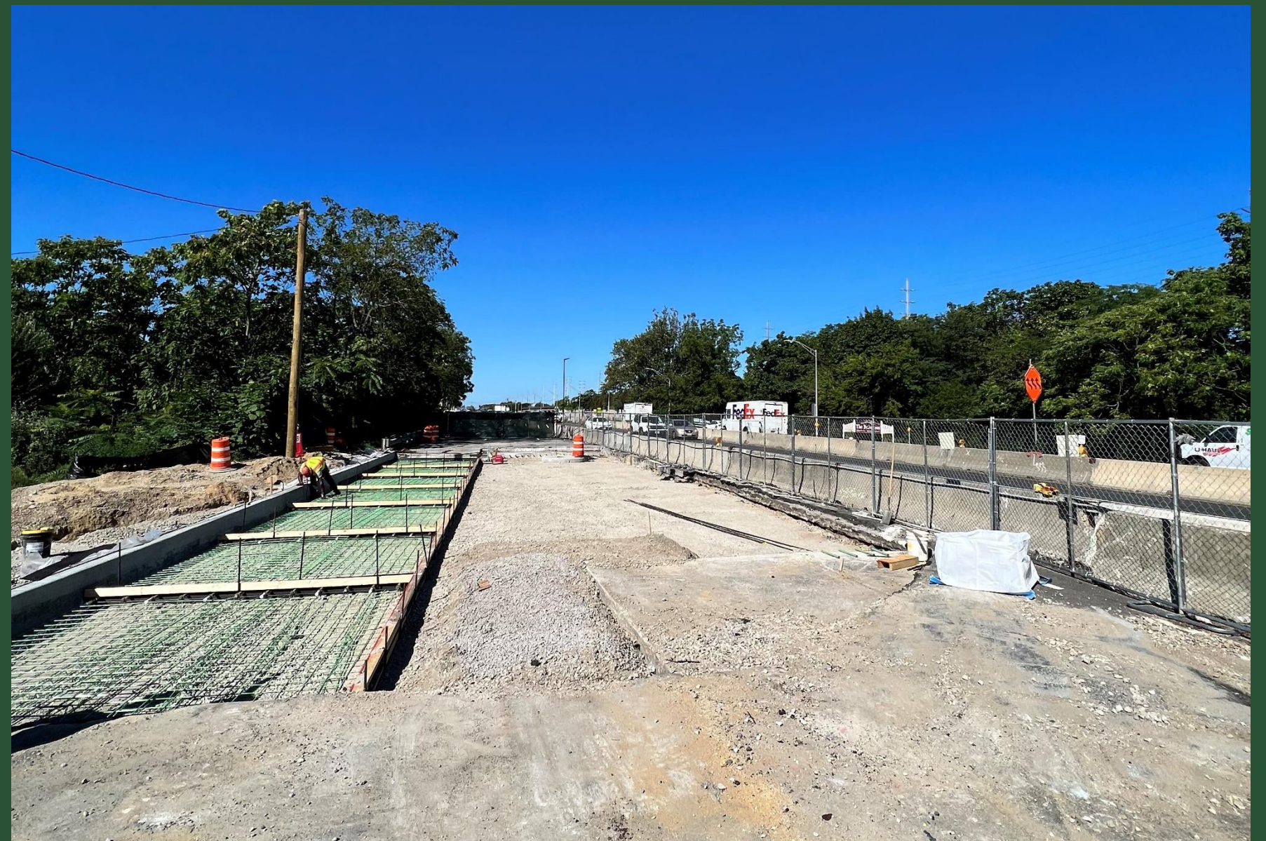
Construction at Pit W (September 2023)
