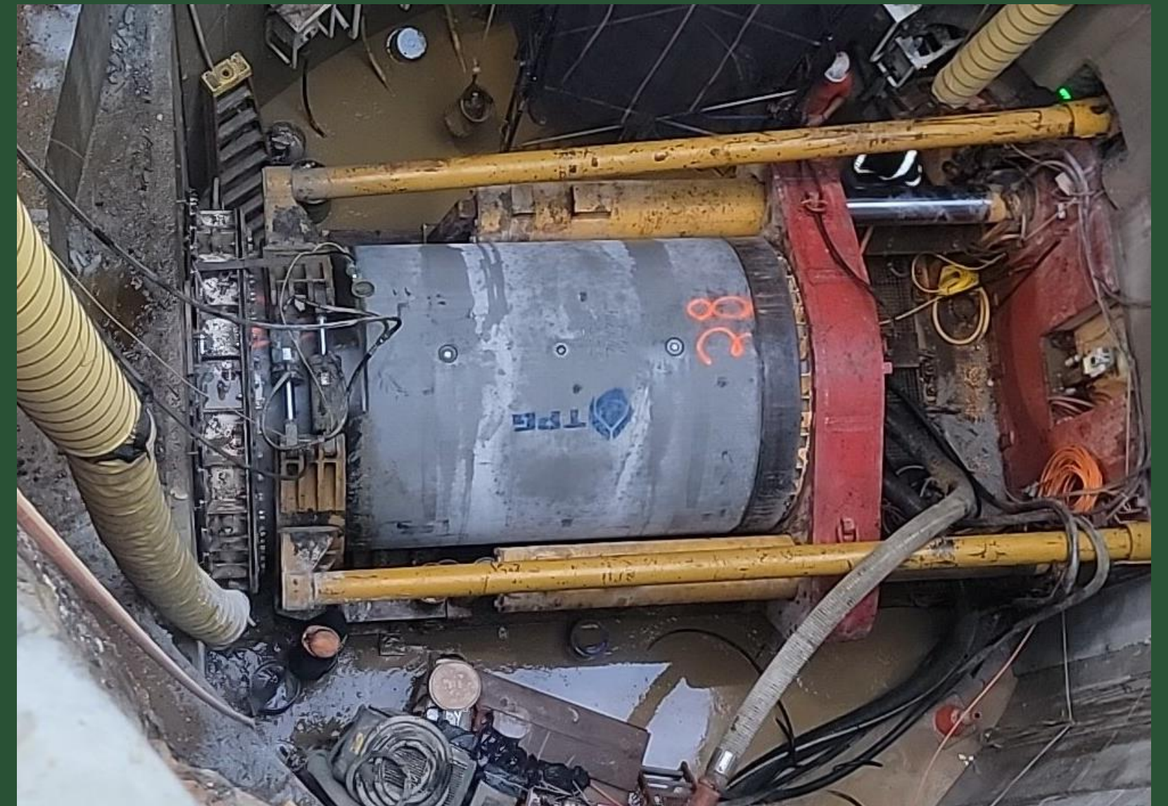
Microtunneling at BP8 (September 2023)
