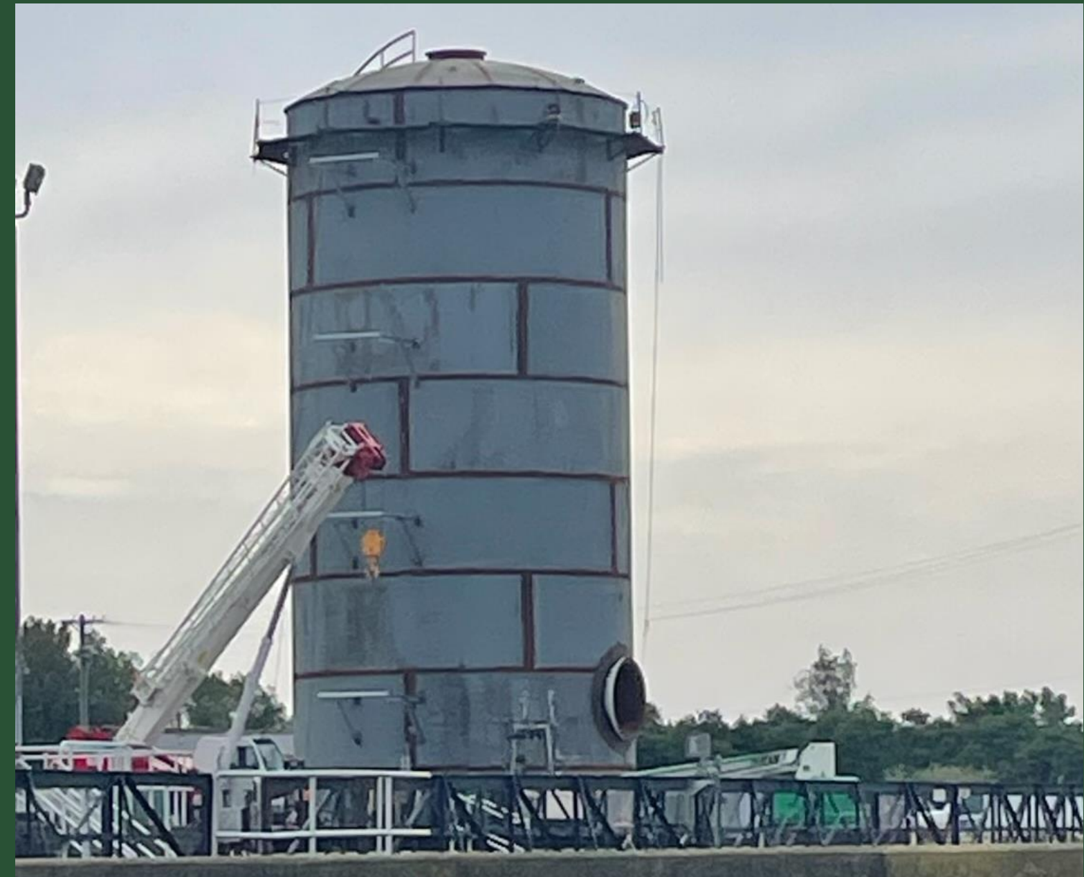
Receiving Tank Structure near CC1 (September 2023)
