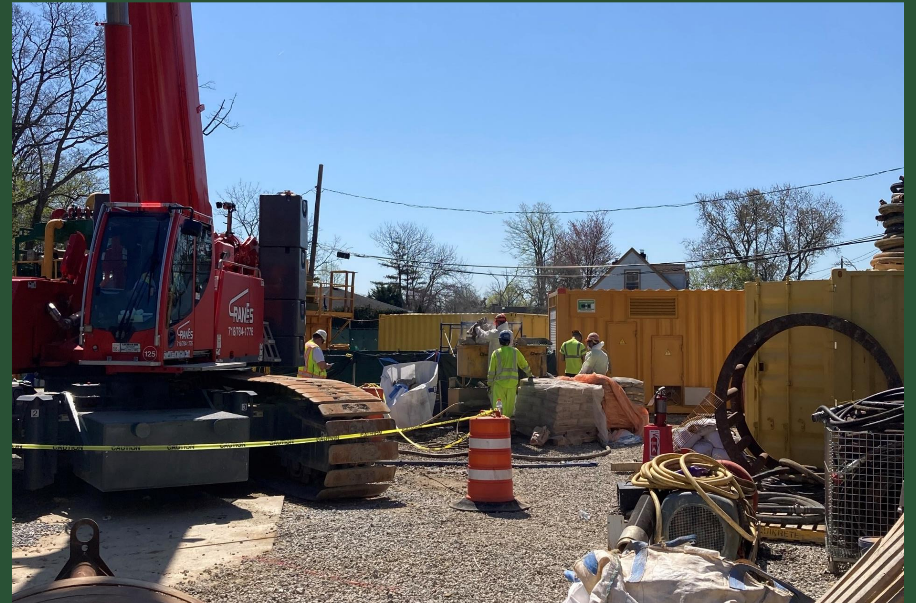
Grouting Activities at CC5 (April 2023)
