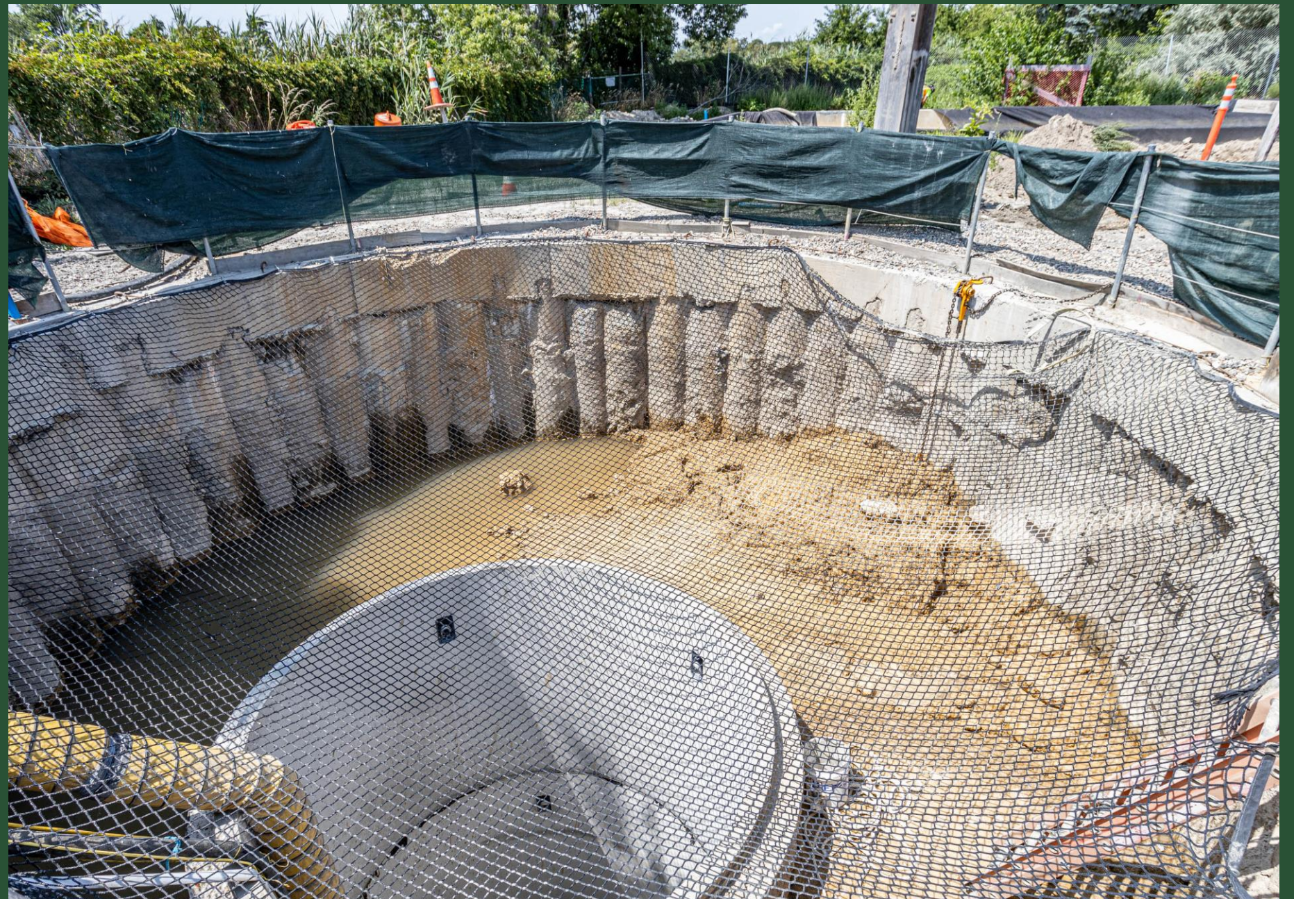
Construction at CC2 (July 2023)
