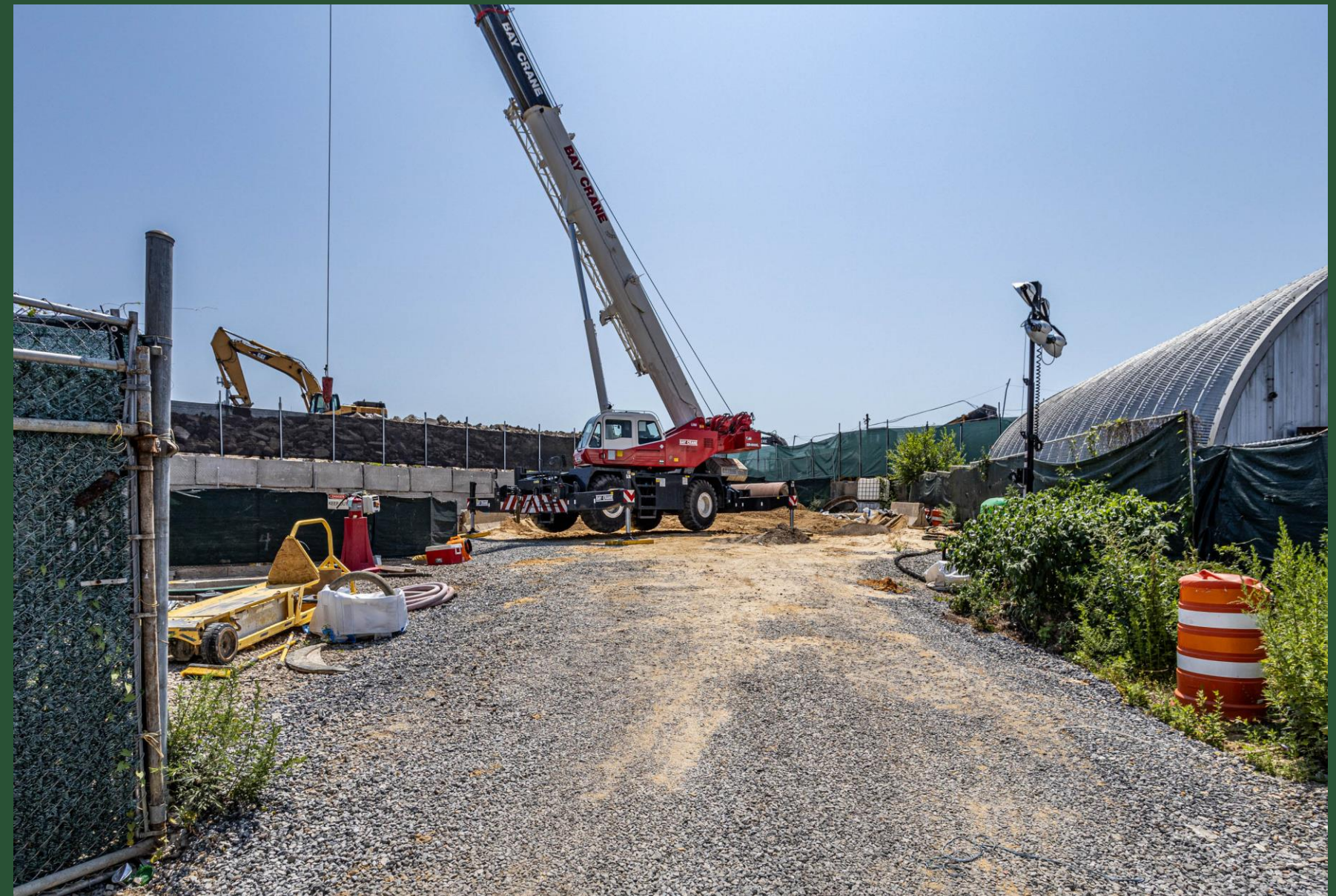
BP3 Restoration Activities (July 2023)
