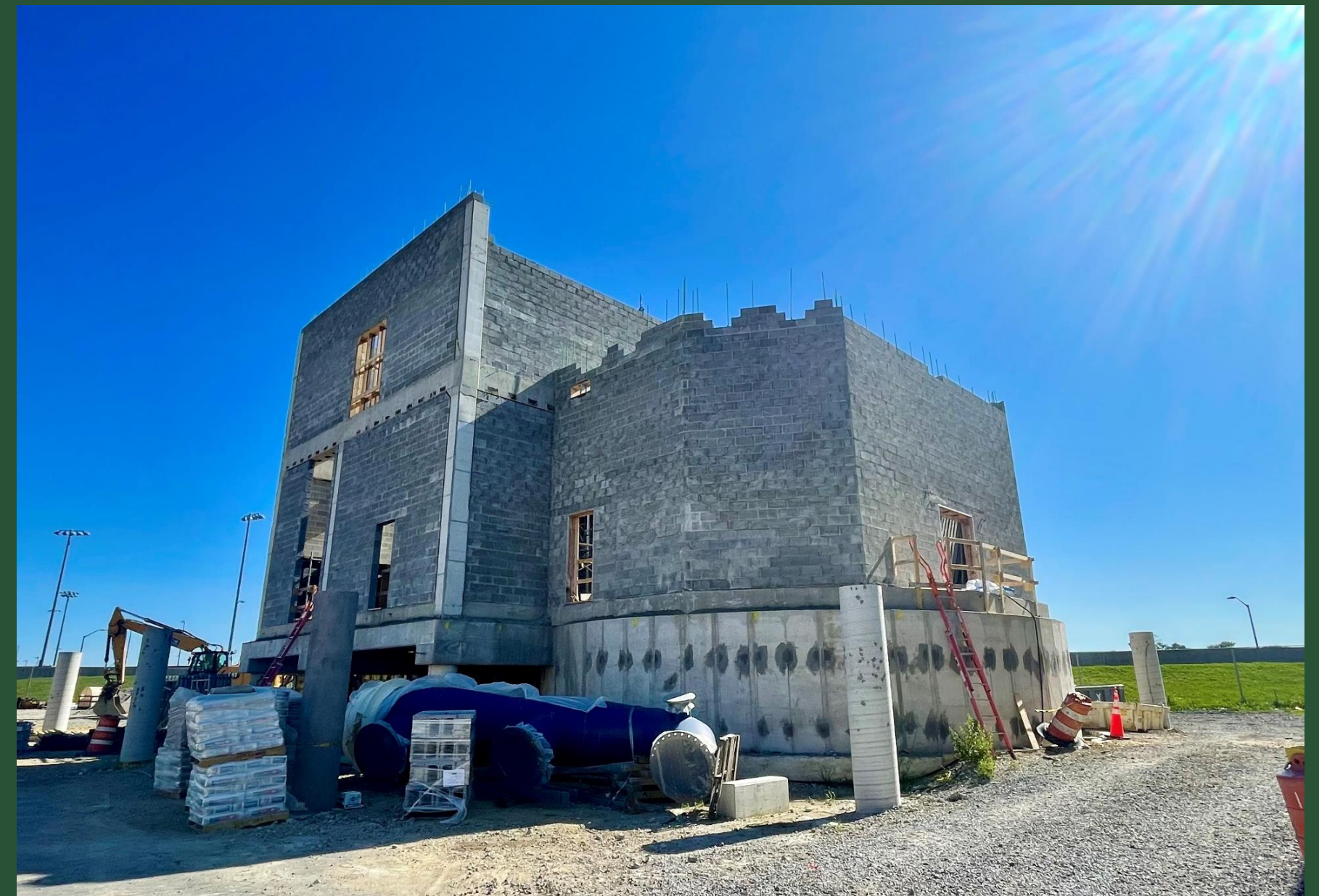
Pump Station Construction Near BP1 (September 2023)
