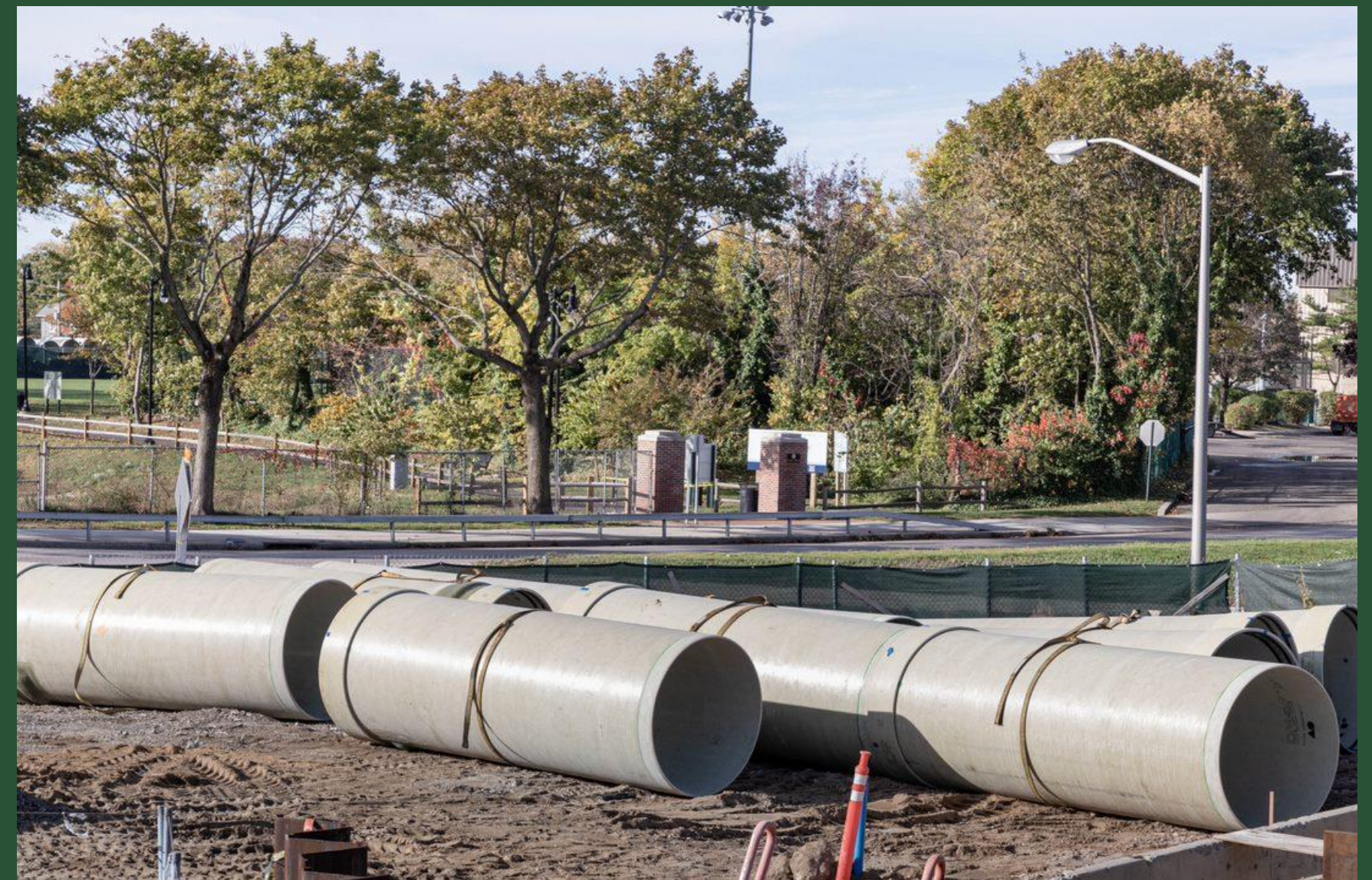
Sliplining Pipe Storage at BP9 (October 2022)
