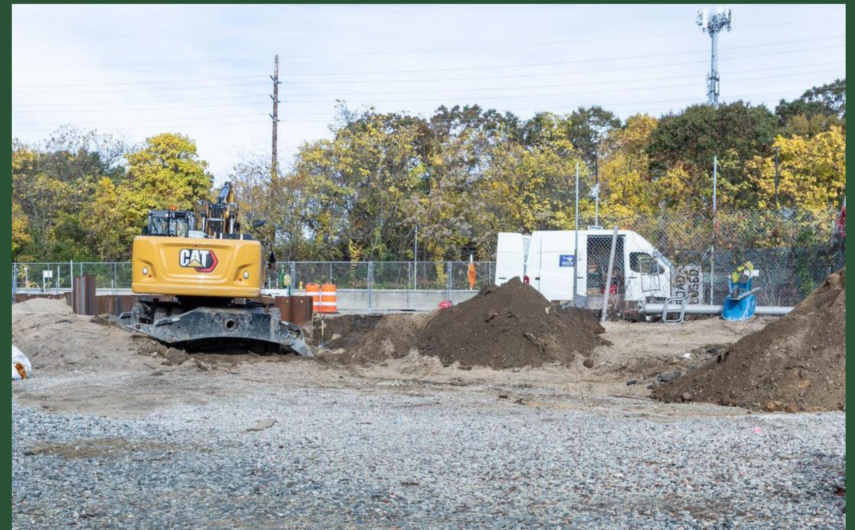
SOE Installation at Pit W (November 2022)
