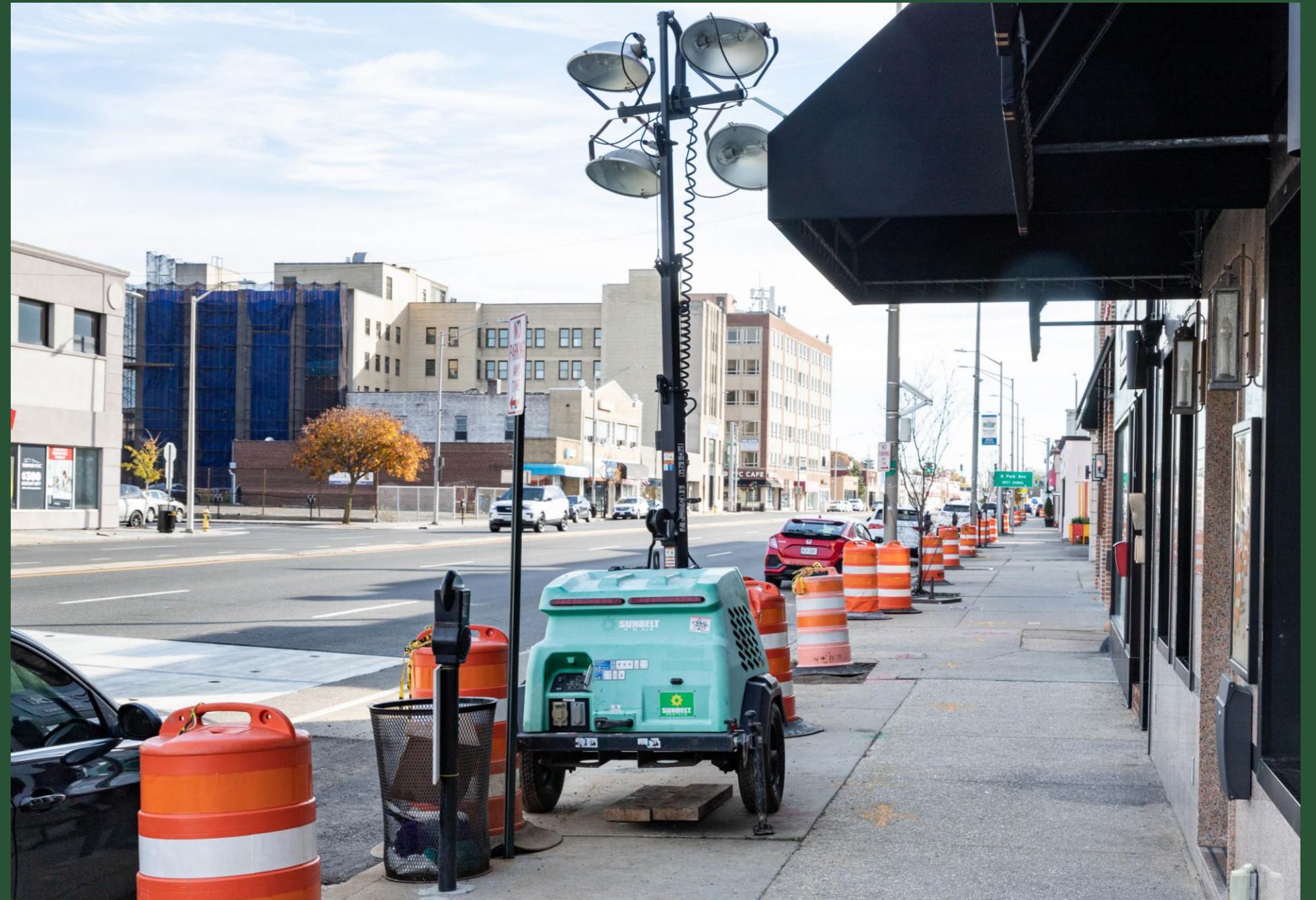
Pit B location on Sunrise Highway in Rockville Centre (October 2022)
