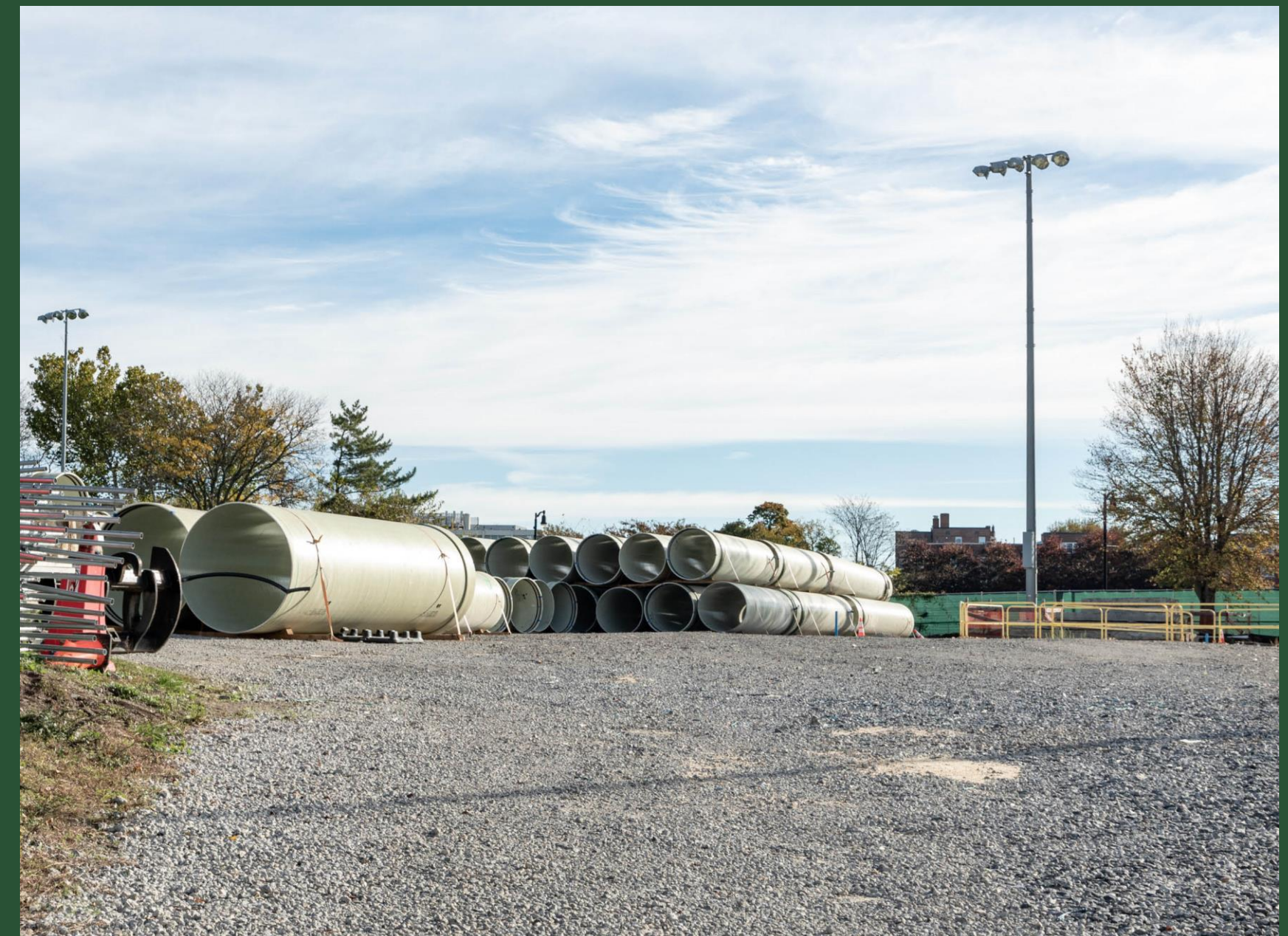
Pipe Storage at BP8 (October 2022)
