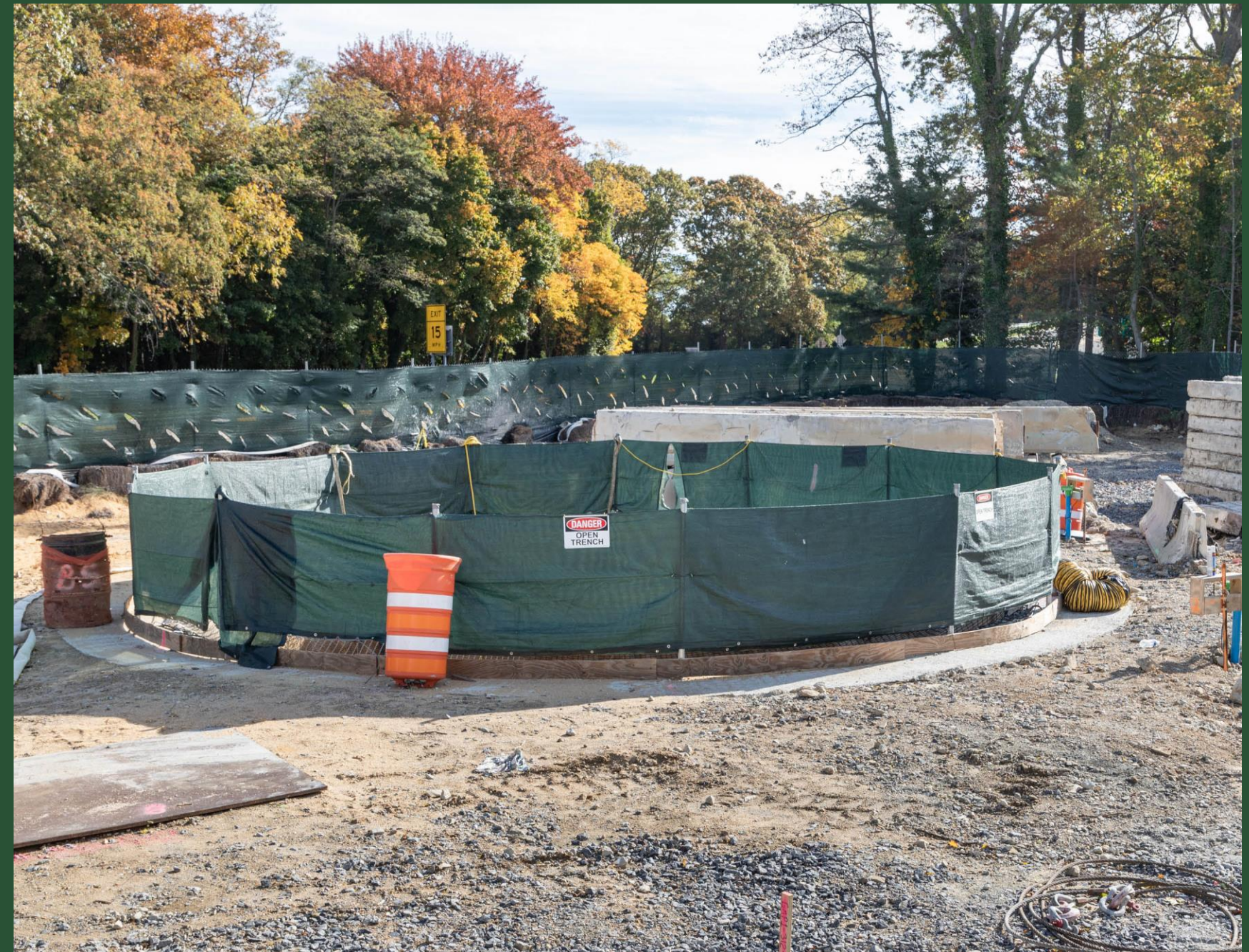
Construction Site at CC5 (July 2022)
