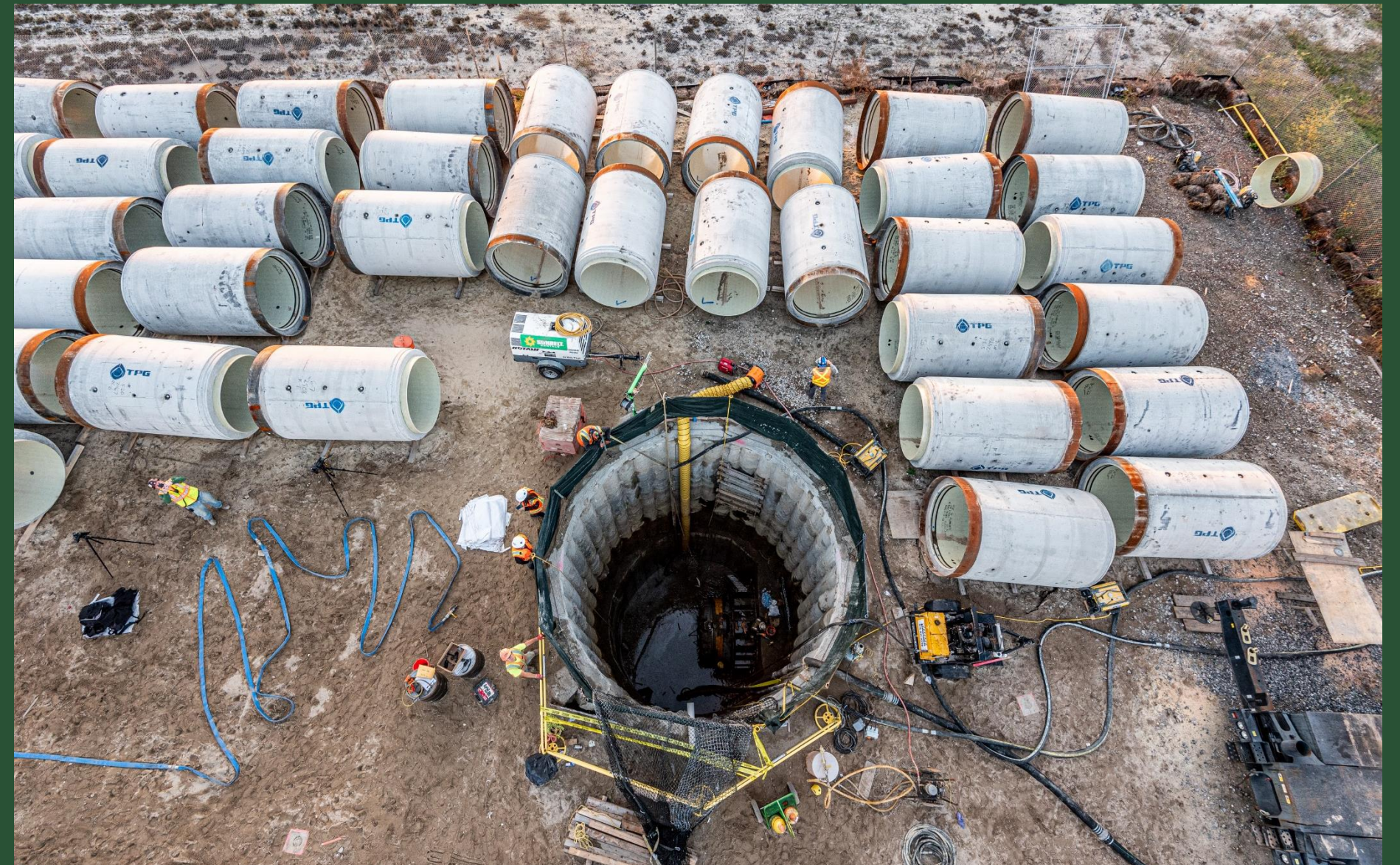
MTBM Breakthrough at CC1 (November 2022)
