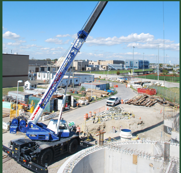
Wet Well Construction near BP1 (September 2022)
