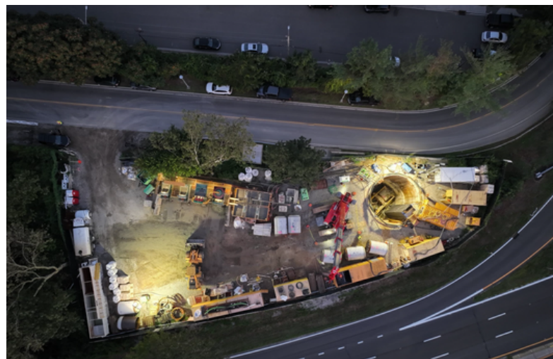
Cedar Creek Shaft 4 Construction Site
