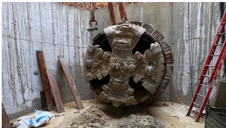
Breakthrough at Bay Park Shaft 9
