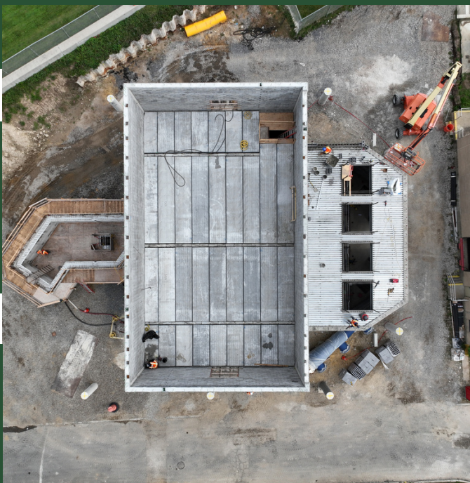
Pump Station Progress
