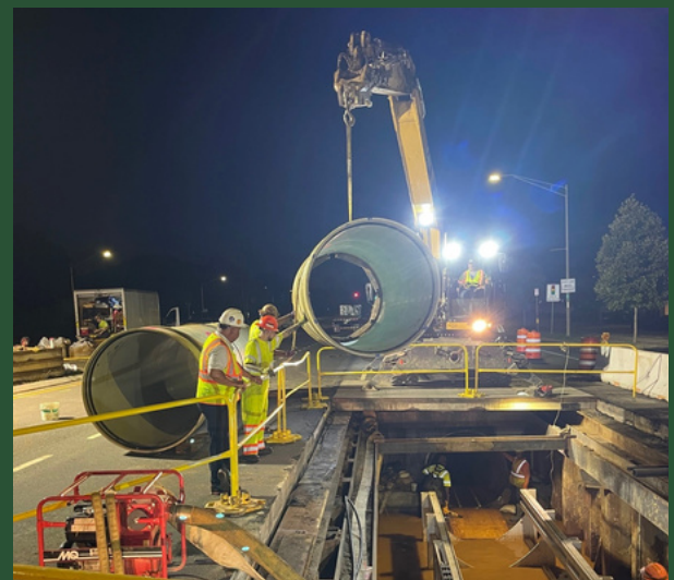
Sliplining at Pit T (July 2022)
