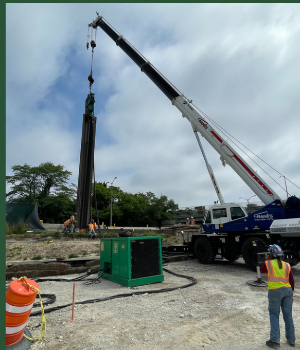
Sheet Pile Installation at Pit A (June 2022)
