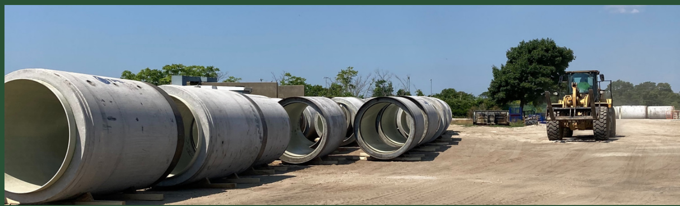
Pipe Delivery at CC1 (July 2022)
