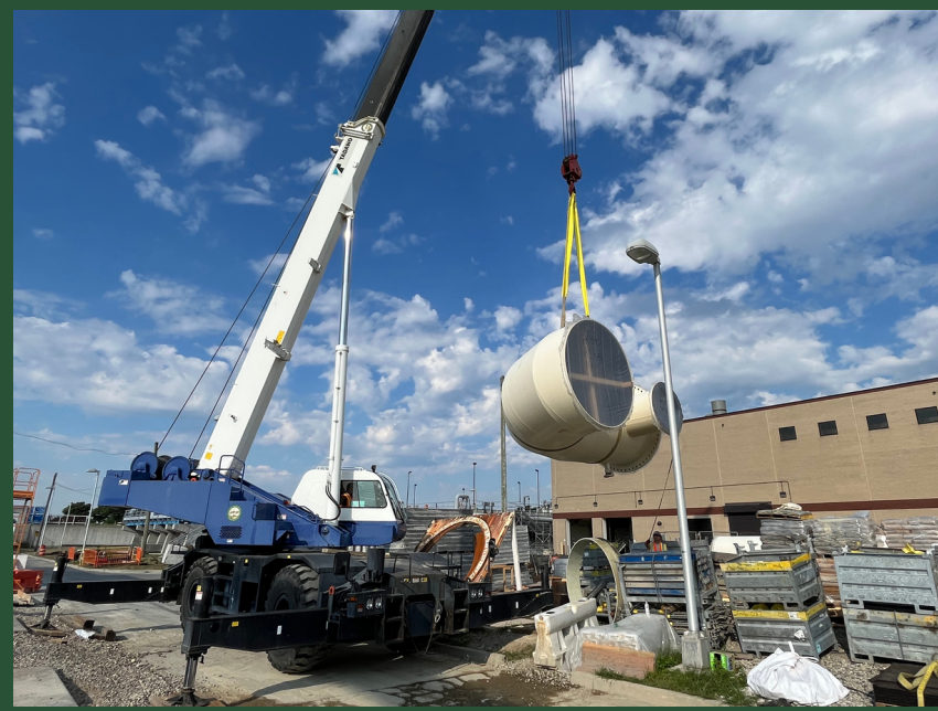
Pipe Installation at BP1 (July 2022)
