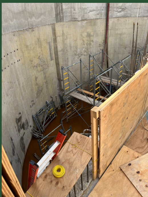
Wet Well Construction at BP1 (July 2022)
