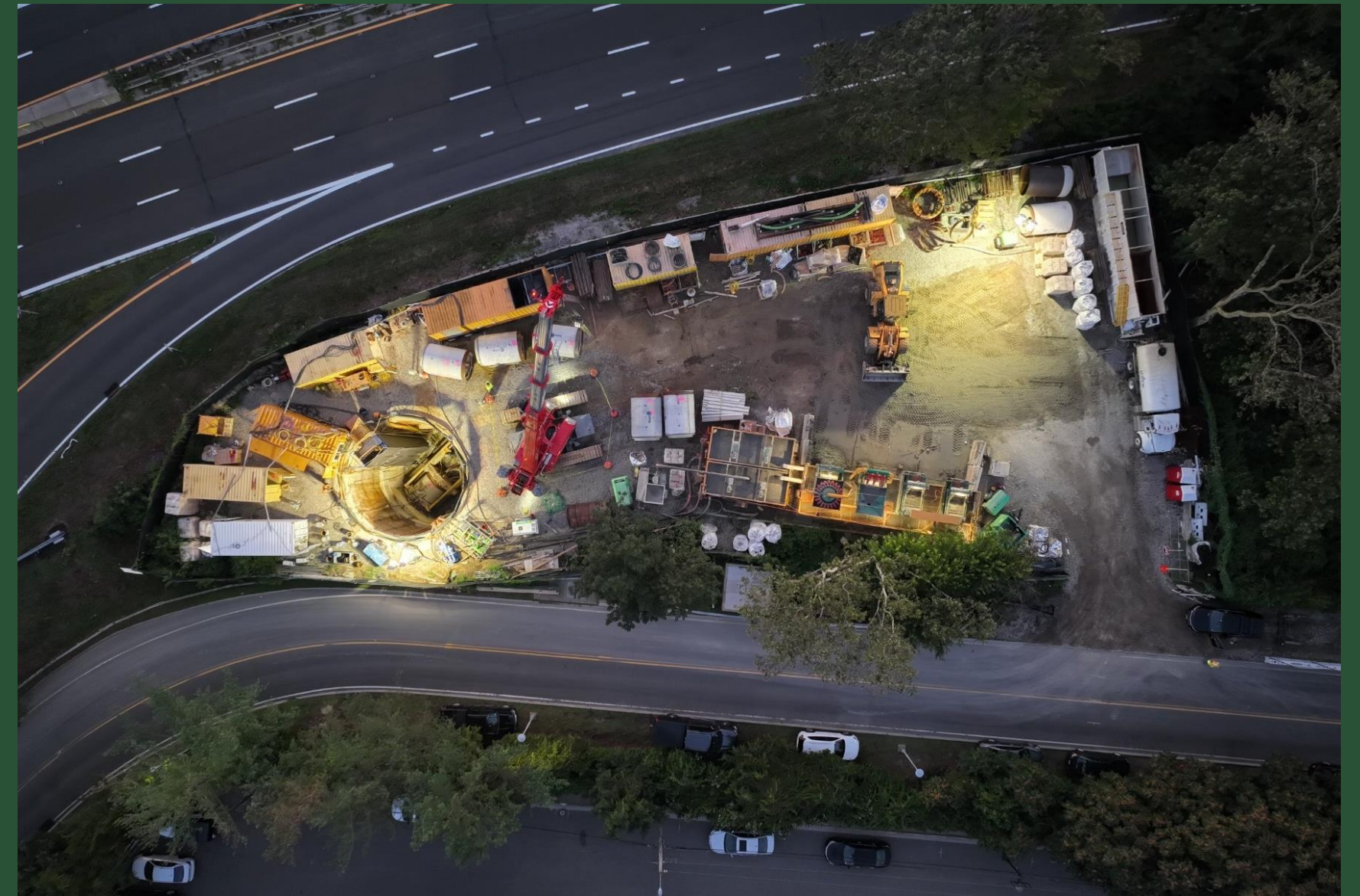
Microtunneling at CC4 (August 2023)
