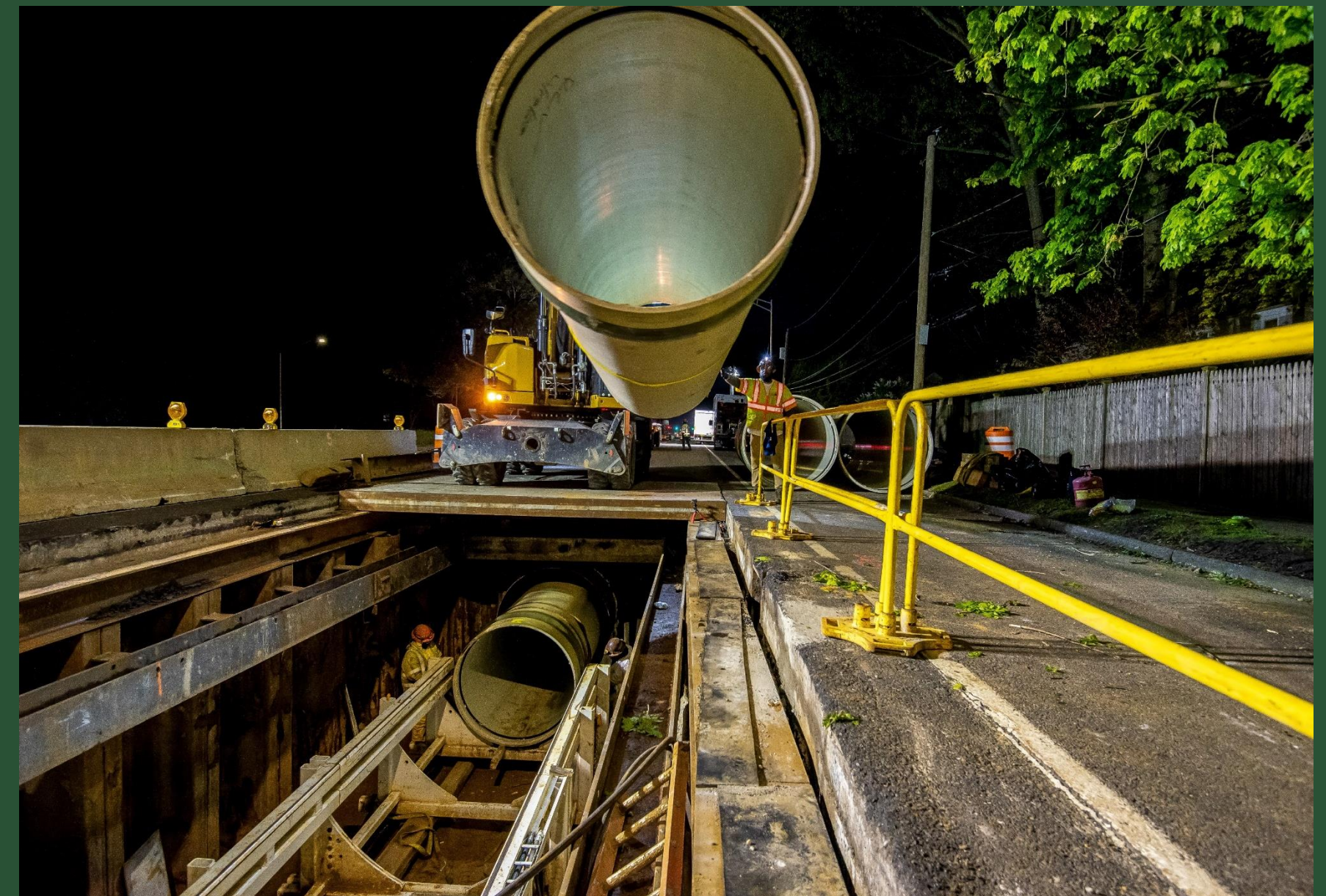
Sliplining at Pit FF (May 2023)
