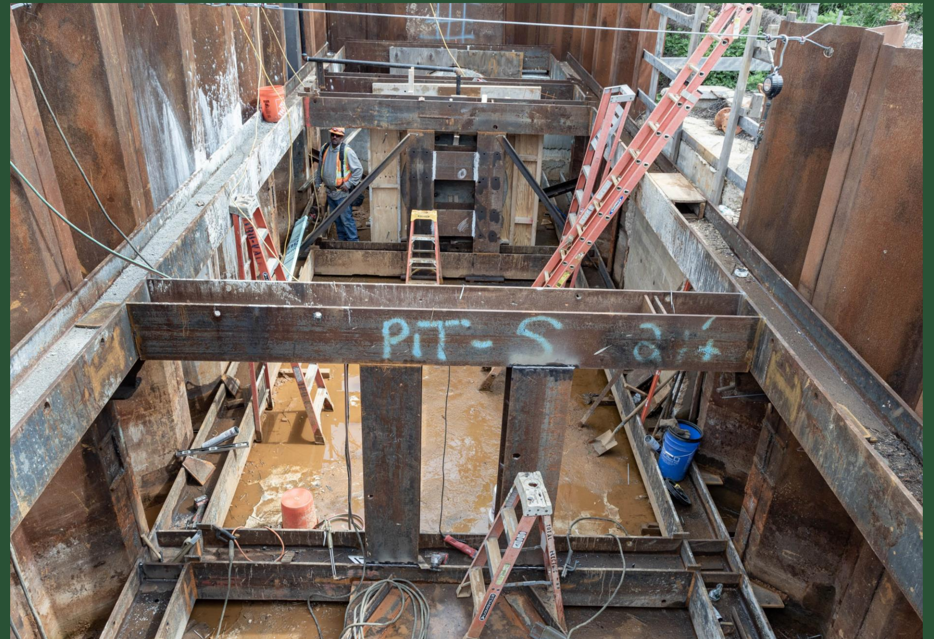
Work at Pit O (April 2023)
