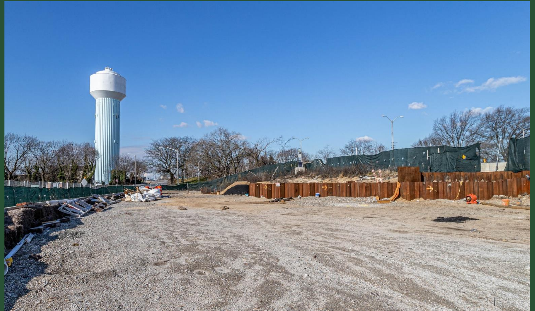
Construction Site at BP9 (January 2023)
