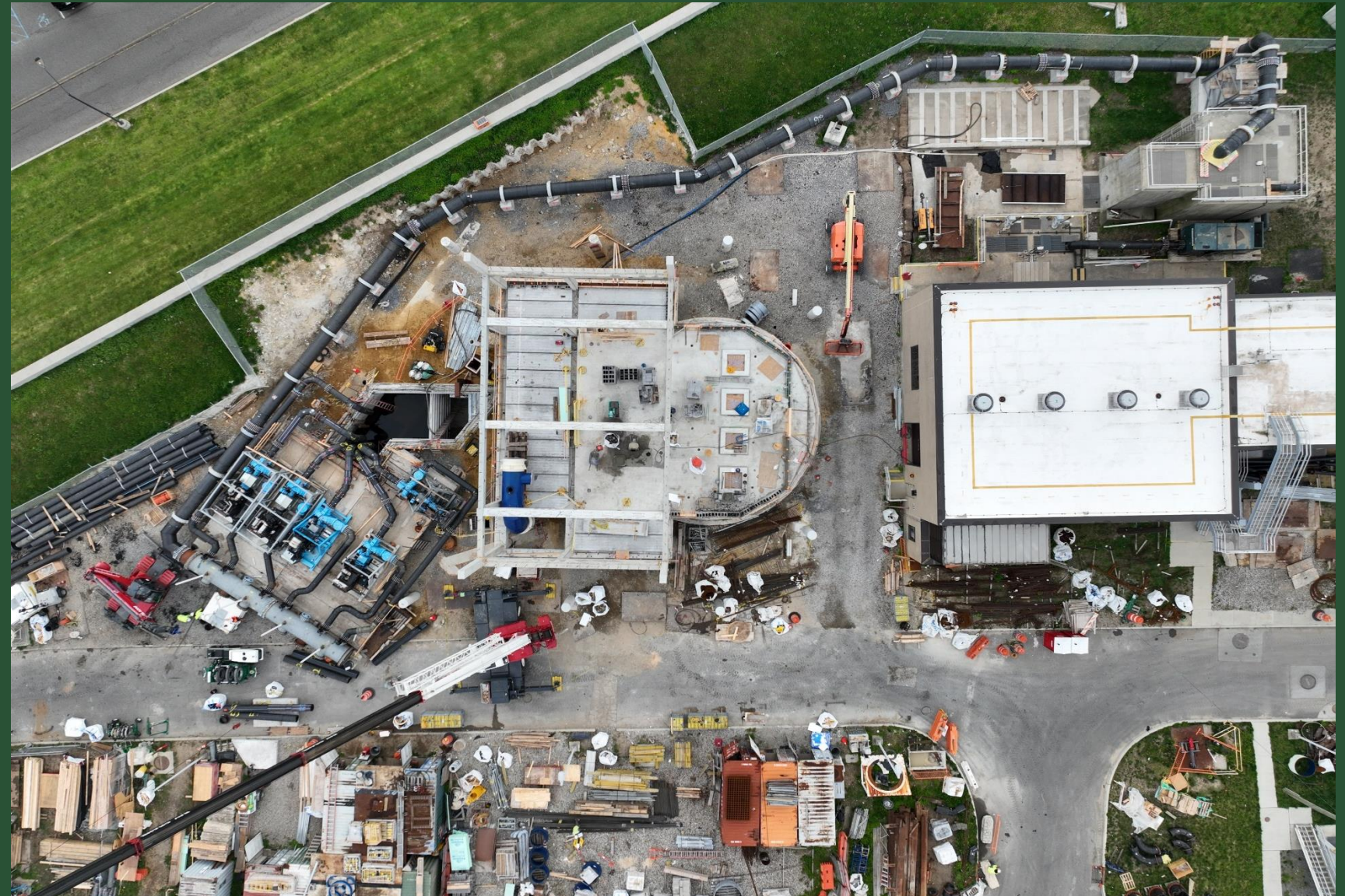
Pump Station Construction Near BP1 (April 2023)
