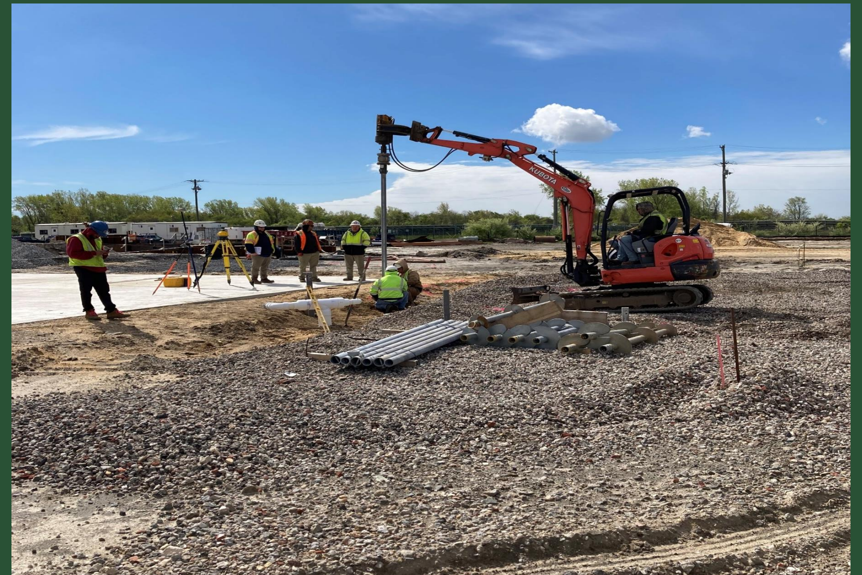
Helical Pile Installation near CC1 (April 2023)
