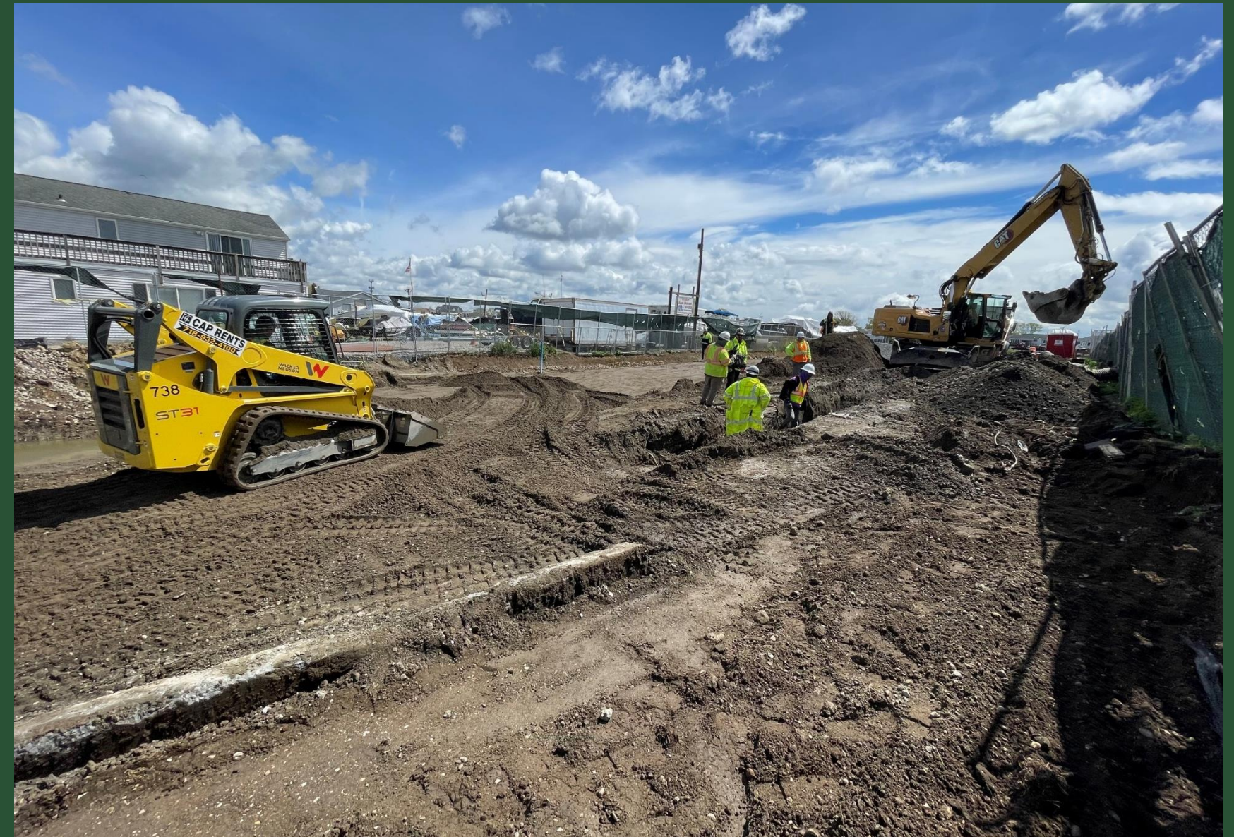
BP2 Restoration Activities (May 2023)
