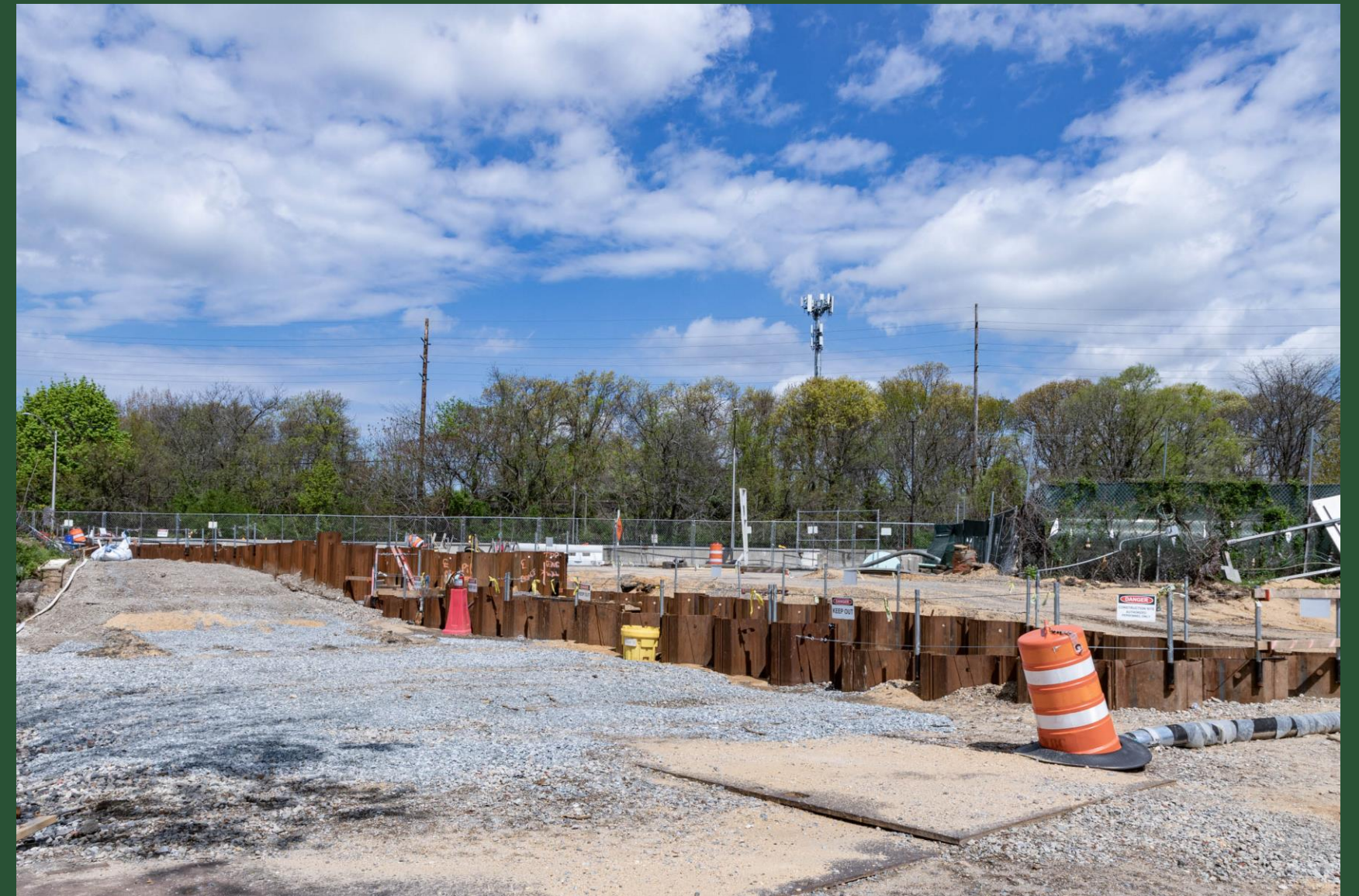
SOE near Pit W (April 2023)
