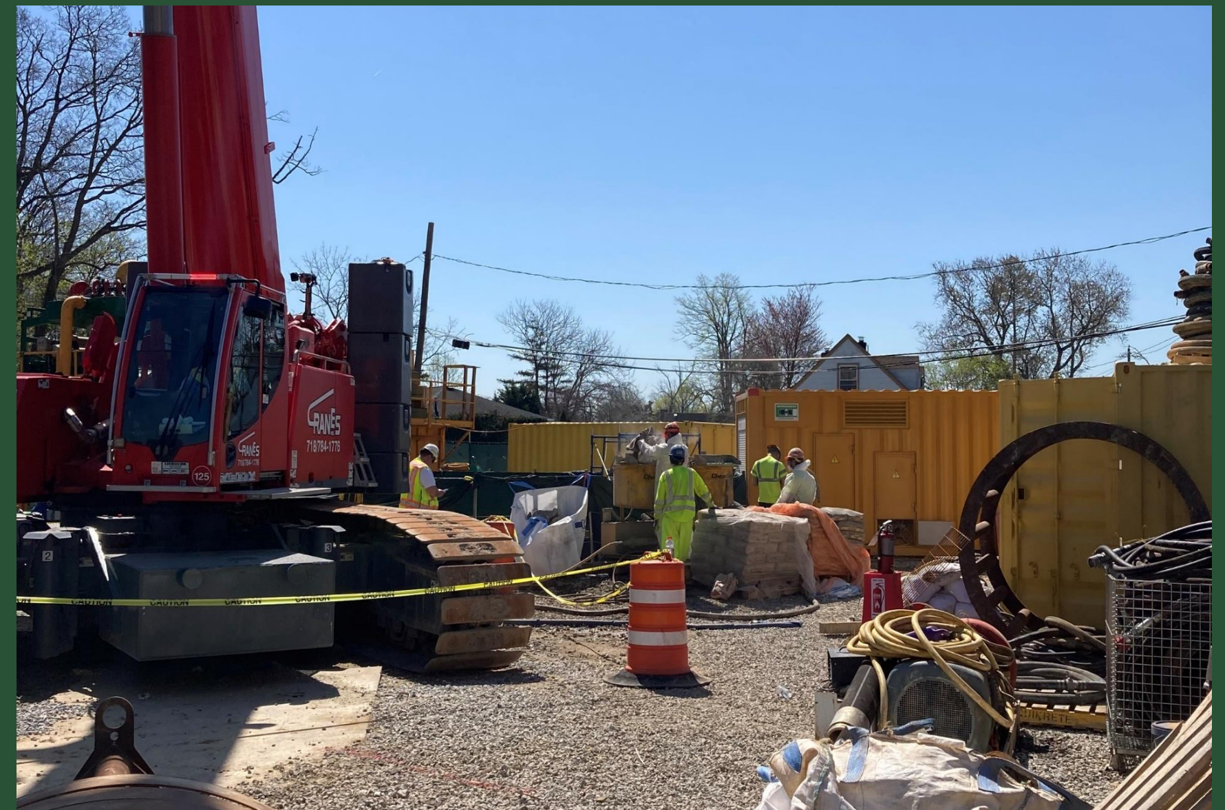
Grouting Activities at CC5 (April 2023)
