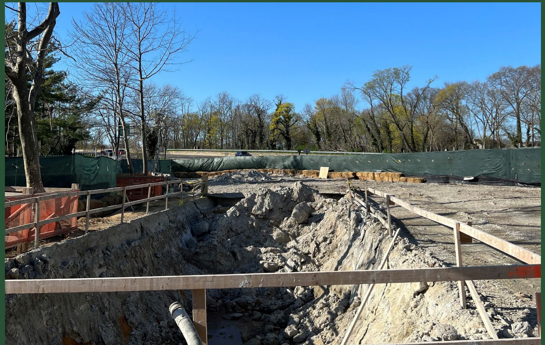
Construction site at CC4 (April 2022)
