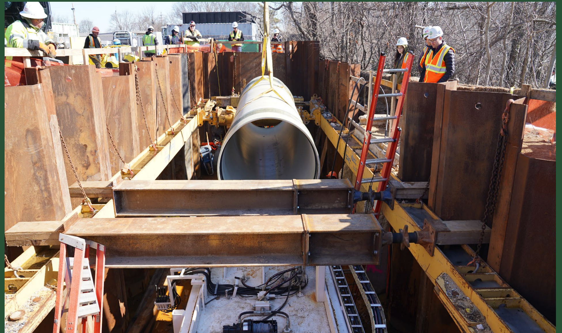
Start of Sliplining at Pit O (March 2022)
