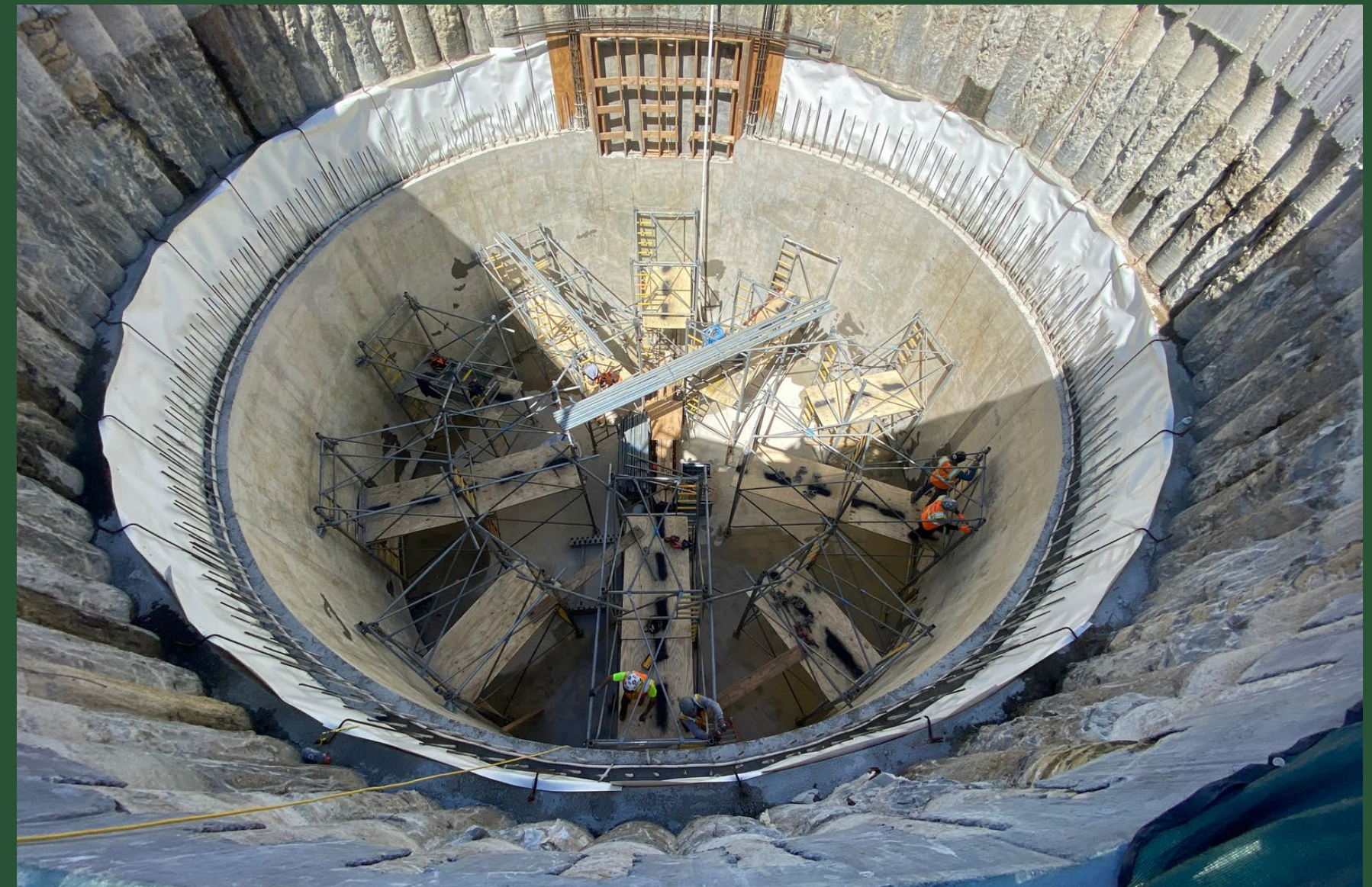
BP1 Wet Well (April 2022)
