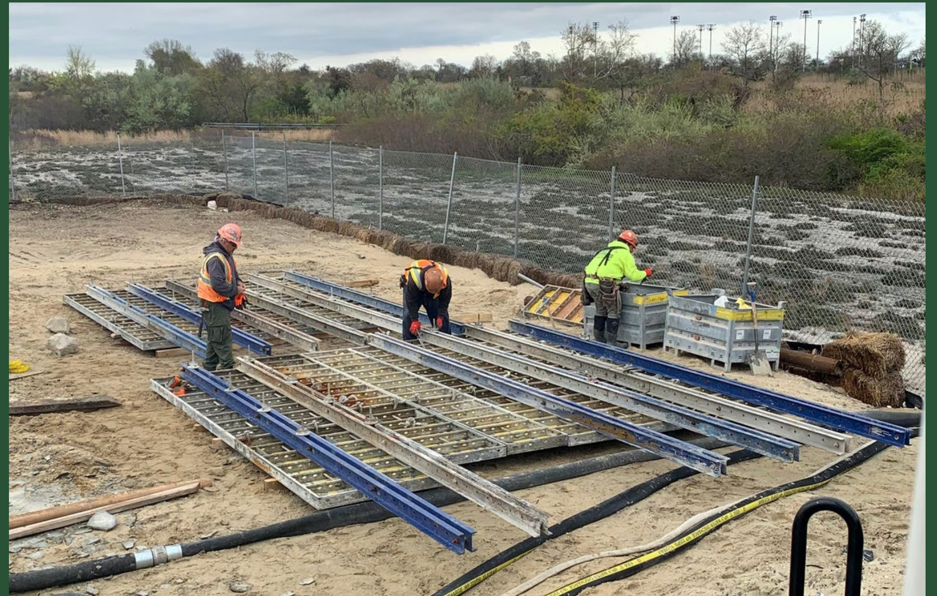
Construction of reinforced concrete liner wall at CC1 (May 2022)
