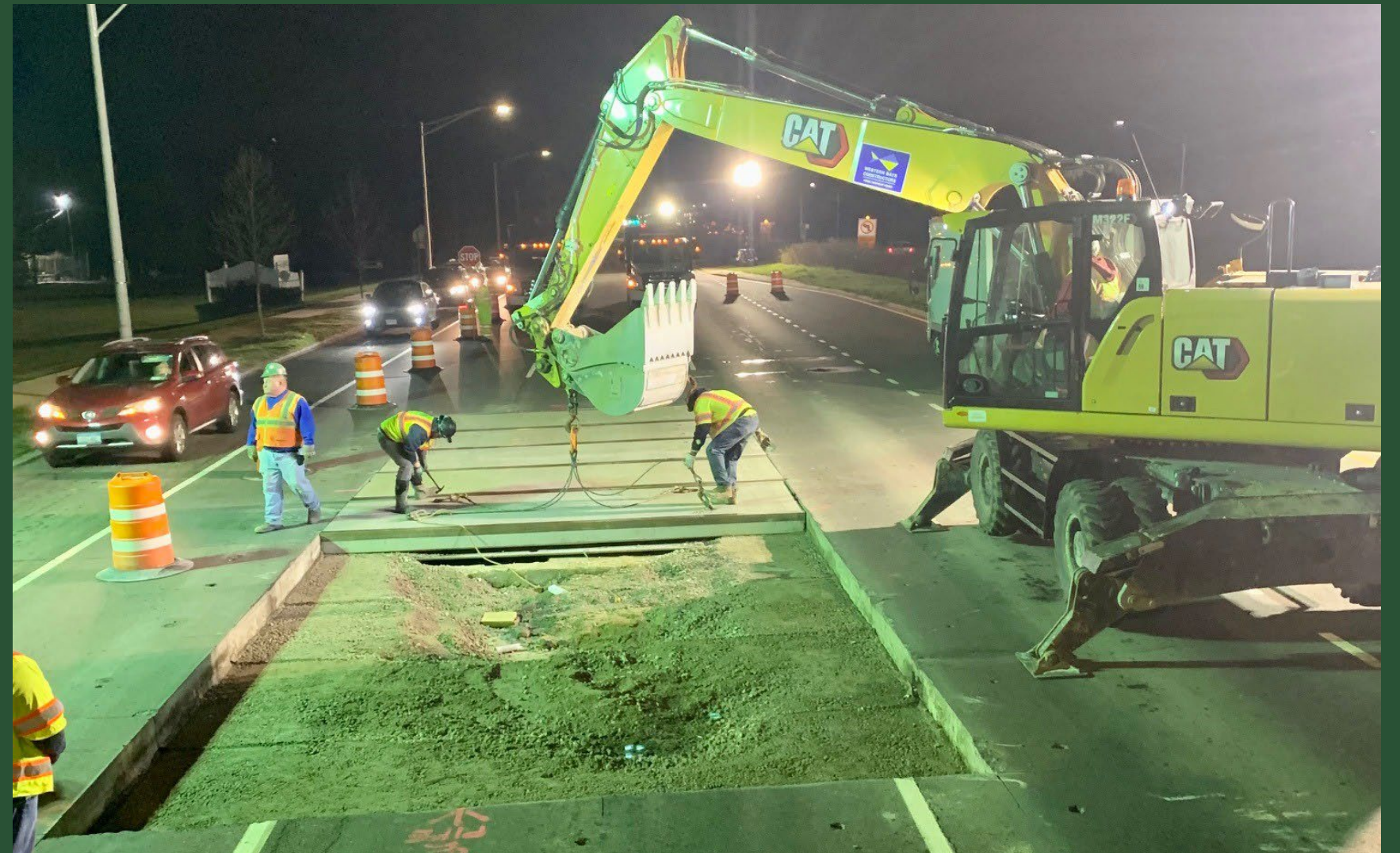
SOE installation at Pit T (April 2022)
