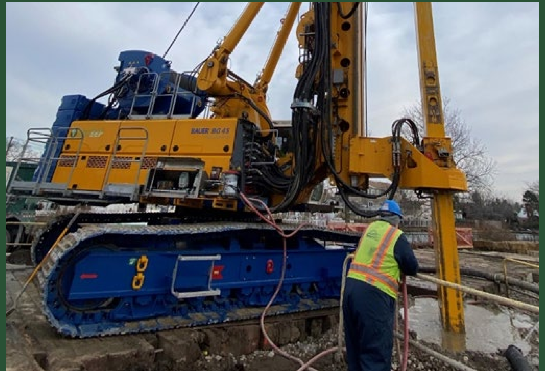
SOE Installation at BP5 (December 2021)
