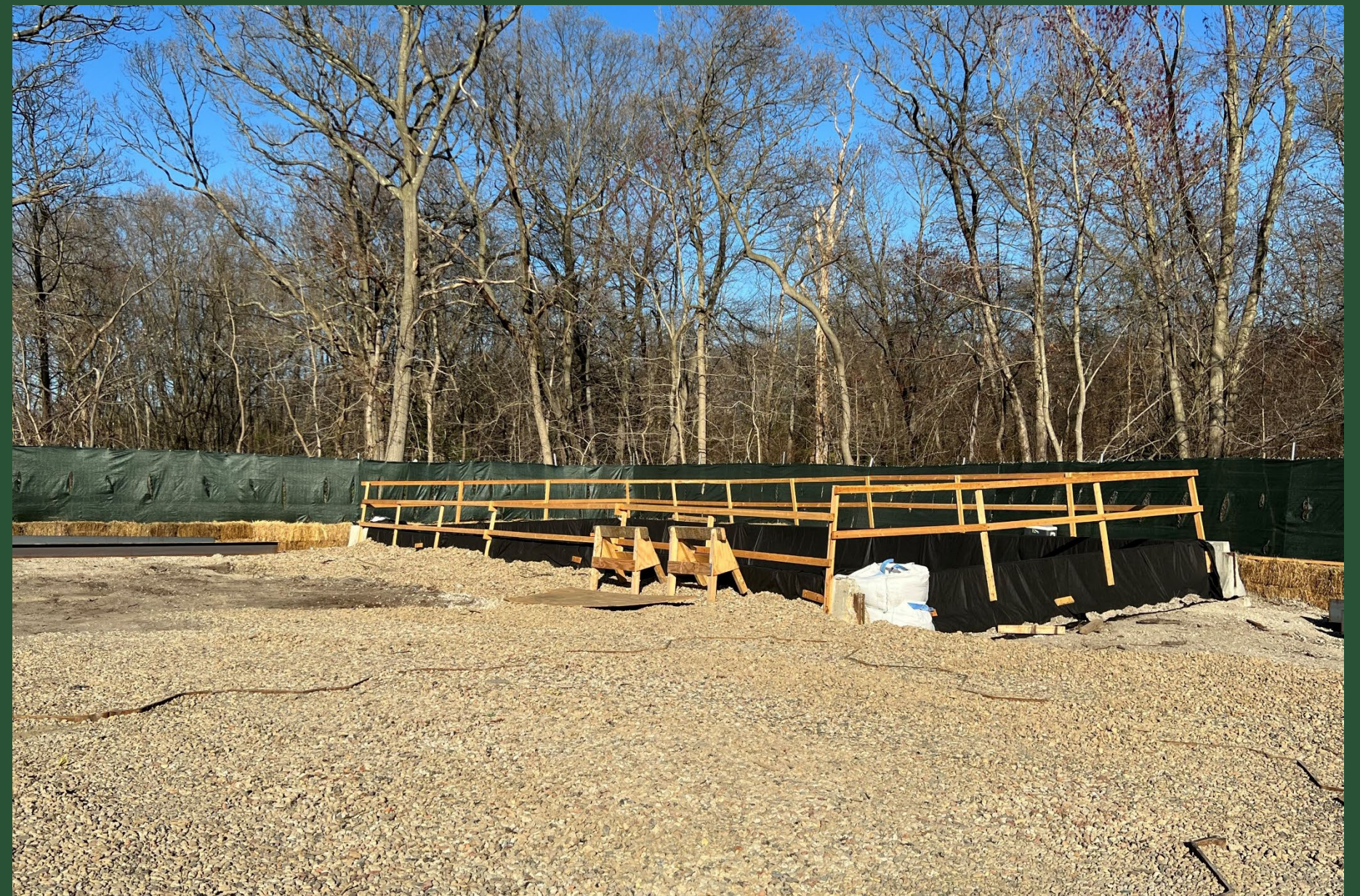
Construction site at CC6 (April 2022)
