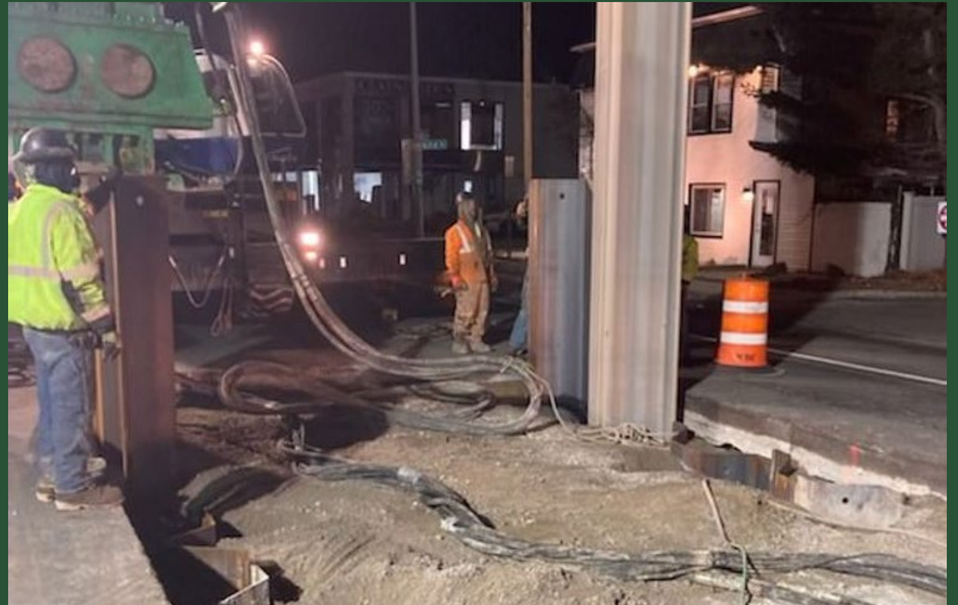
Sheeting installation at Pit R (January 2022)
