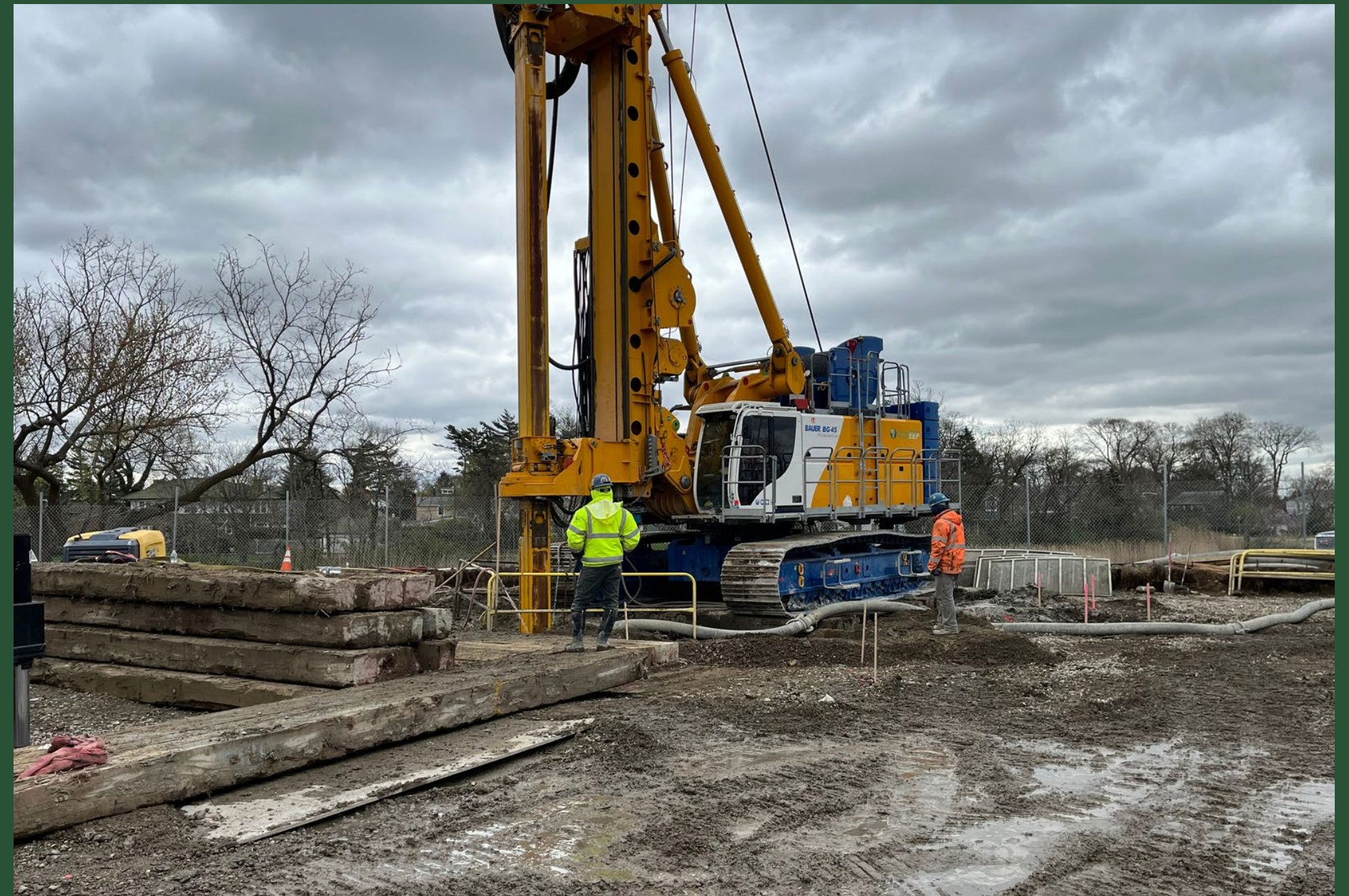
SOE Installation at BP7 (April 2022)
