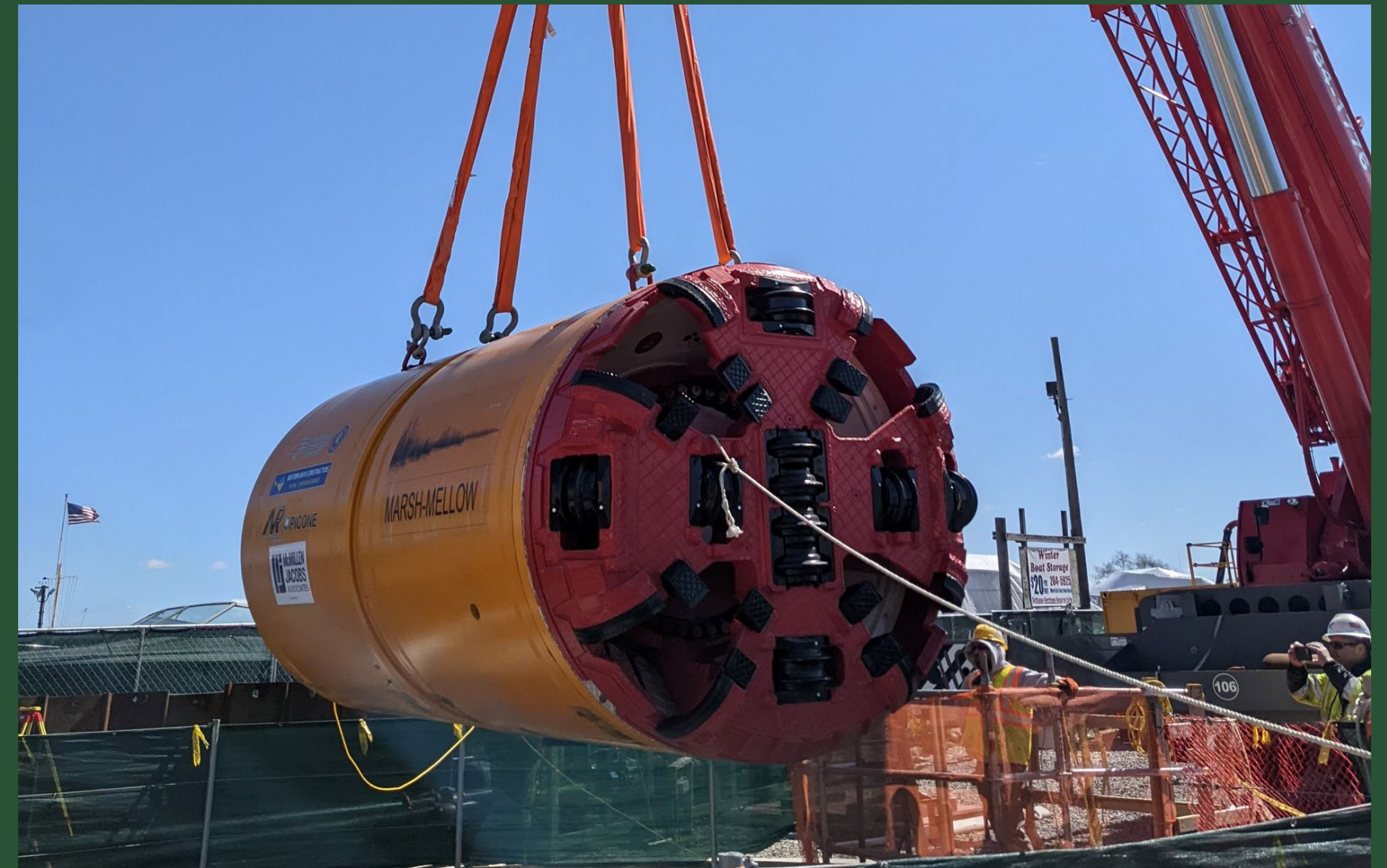
MTBM "MARSH-MELLOW" lowered into BP2 (April 2022)
