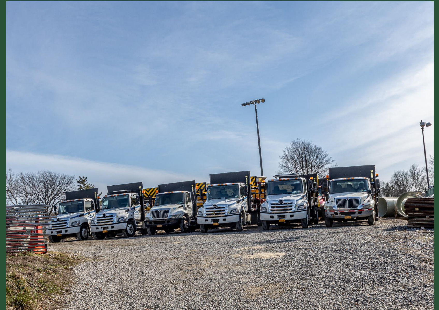
Storage and Laydown at BP8 (February 2023)
