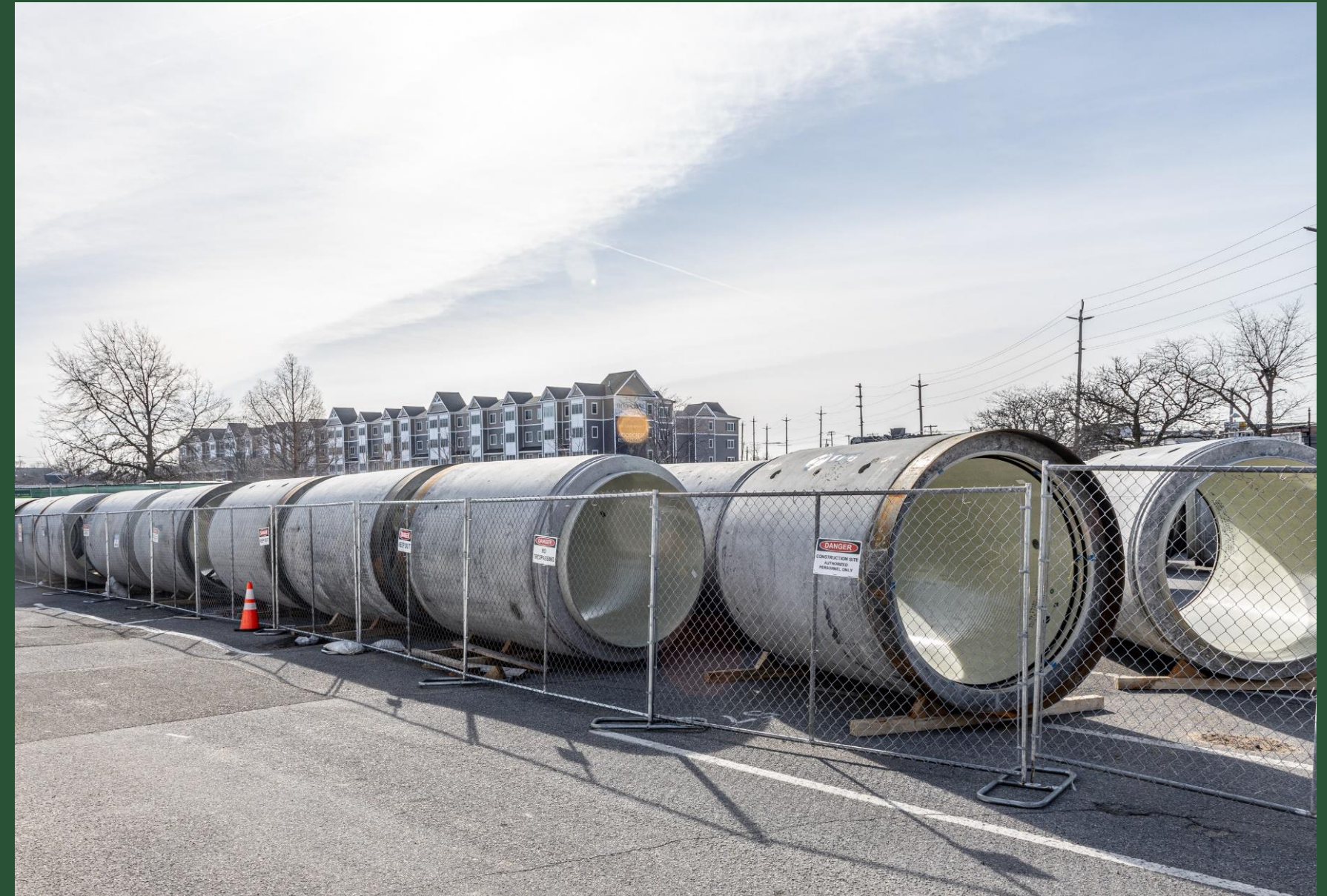
Pipe Storage near BP5 (February 2023)
