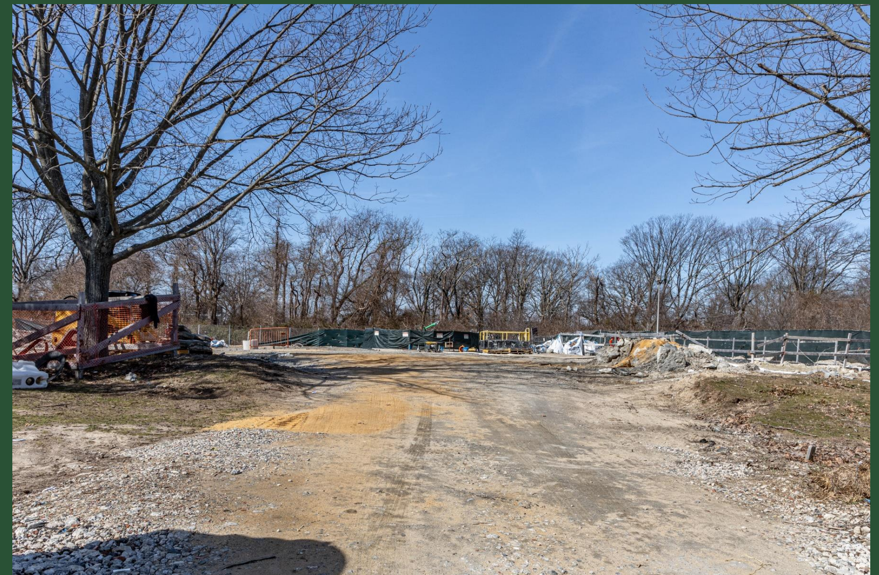
Construction Site at CC3 (February 2023)
