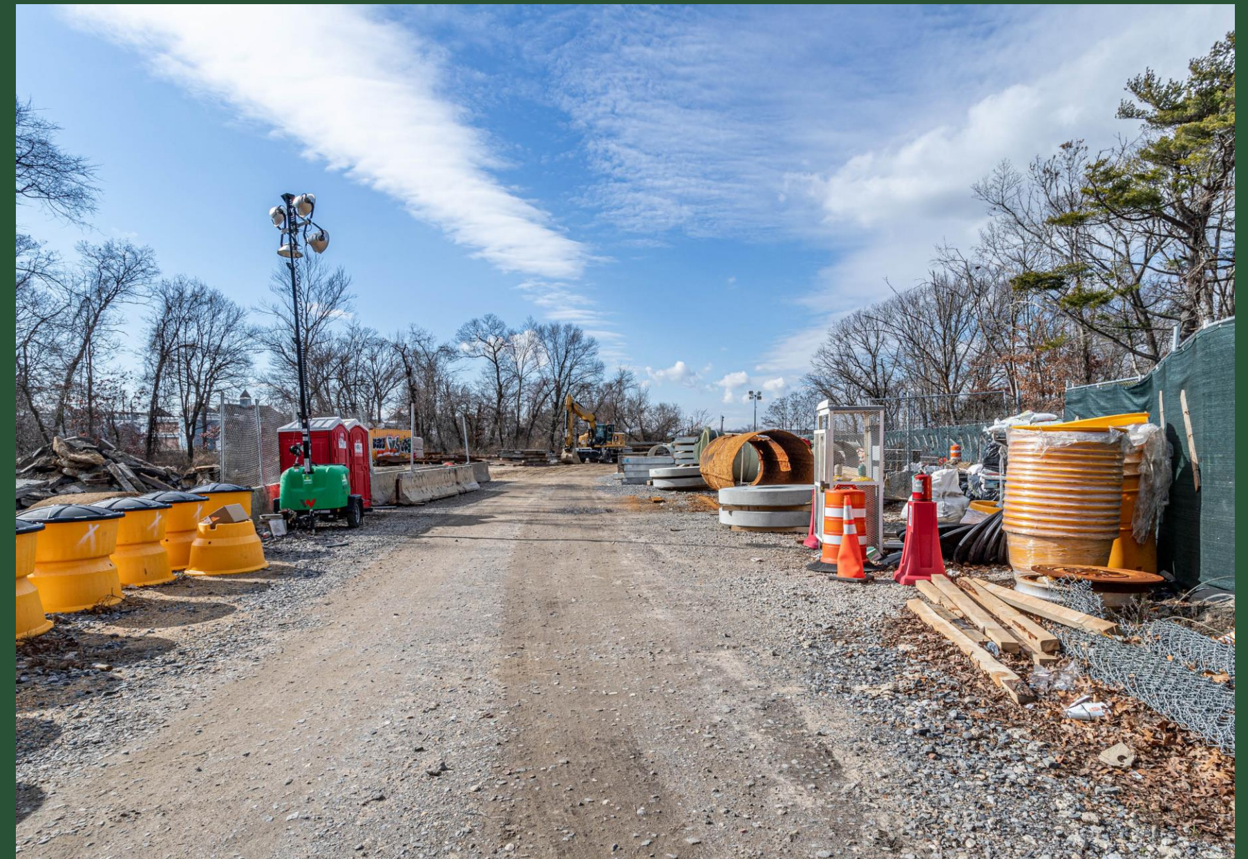
Pit P Construction Site (January 2023)
