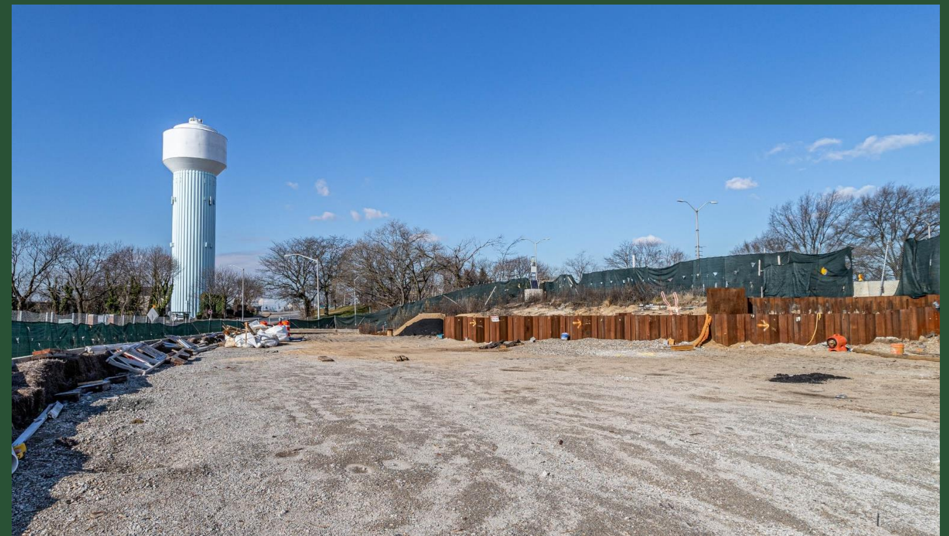
Construction Site at BP9 (January 2023)
