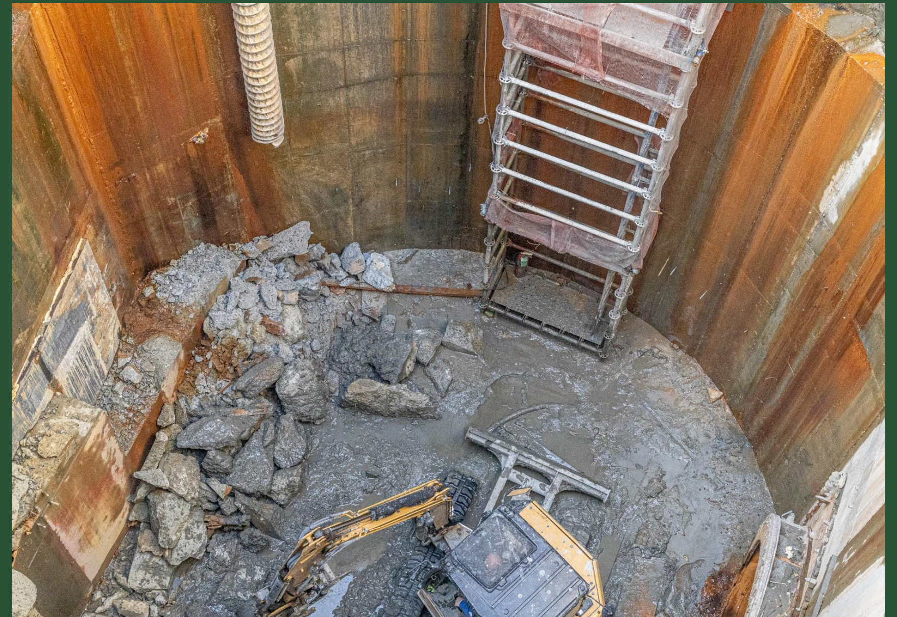
Post Microtunneling Activities at CC2 (February 2023)
