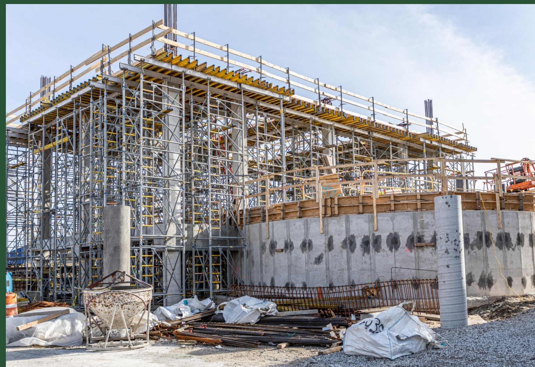
Pump Station Construction Near BP1 (February 2023)
