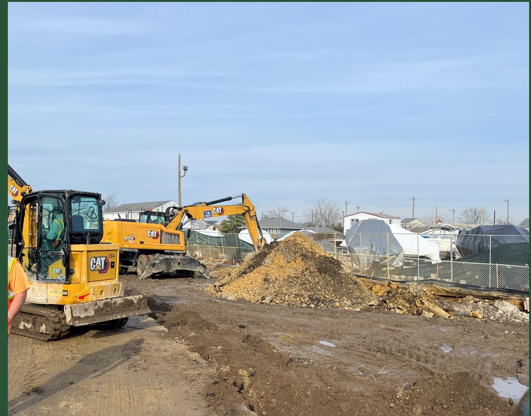
Grading at BP2 (January 2023)
