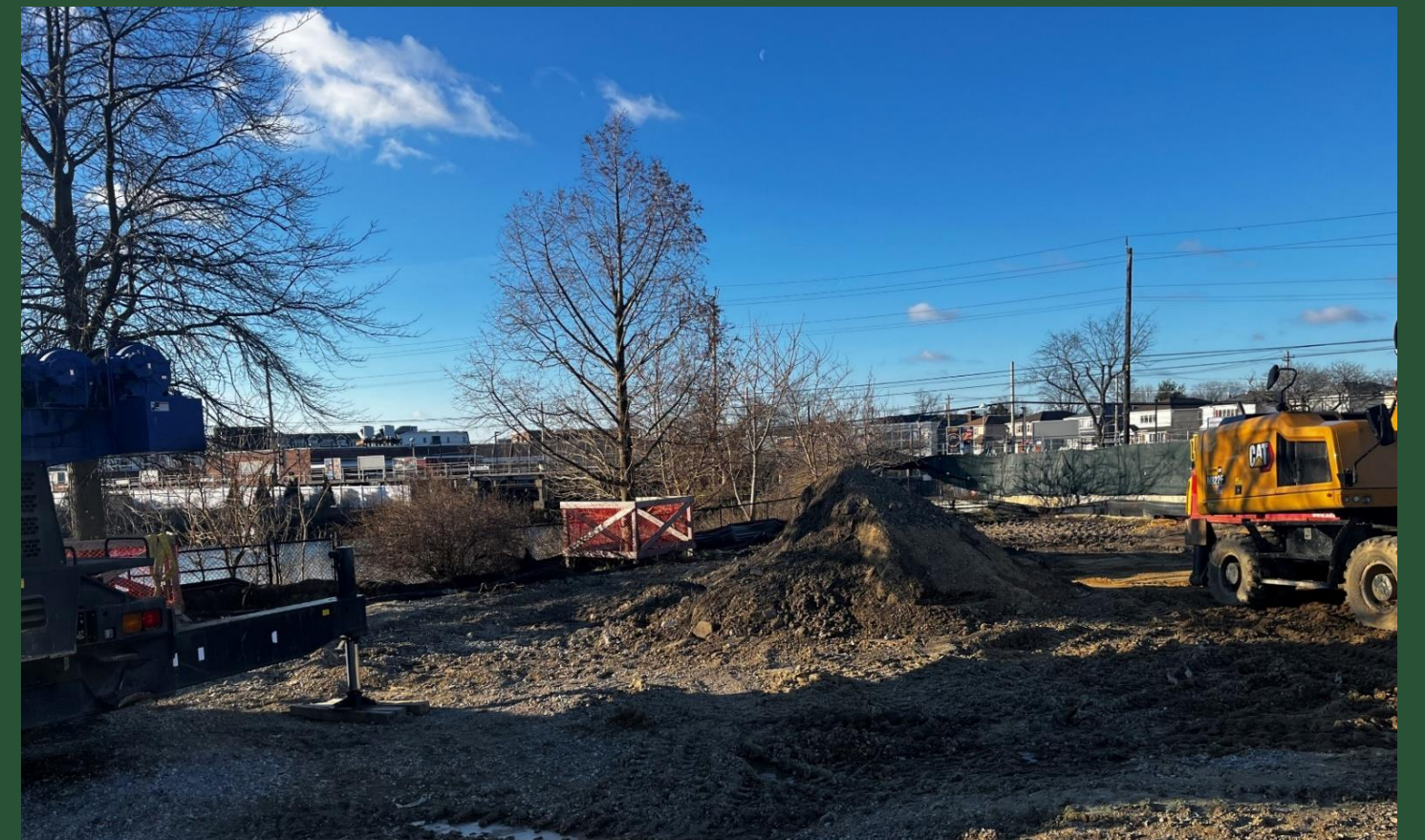
Bay Park Shaft 4 Restoration Activities (December 2023)
