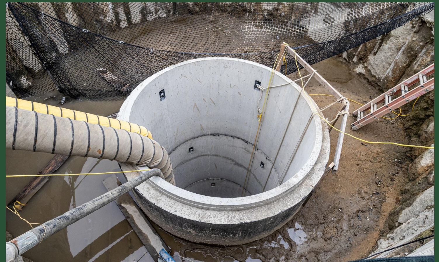
CC2 Manhole Construction (December 2023)
