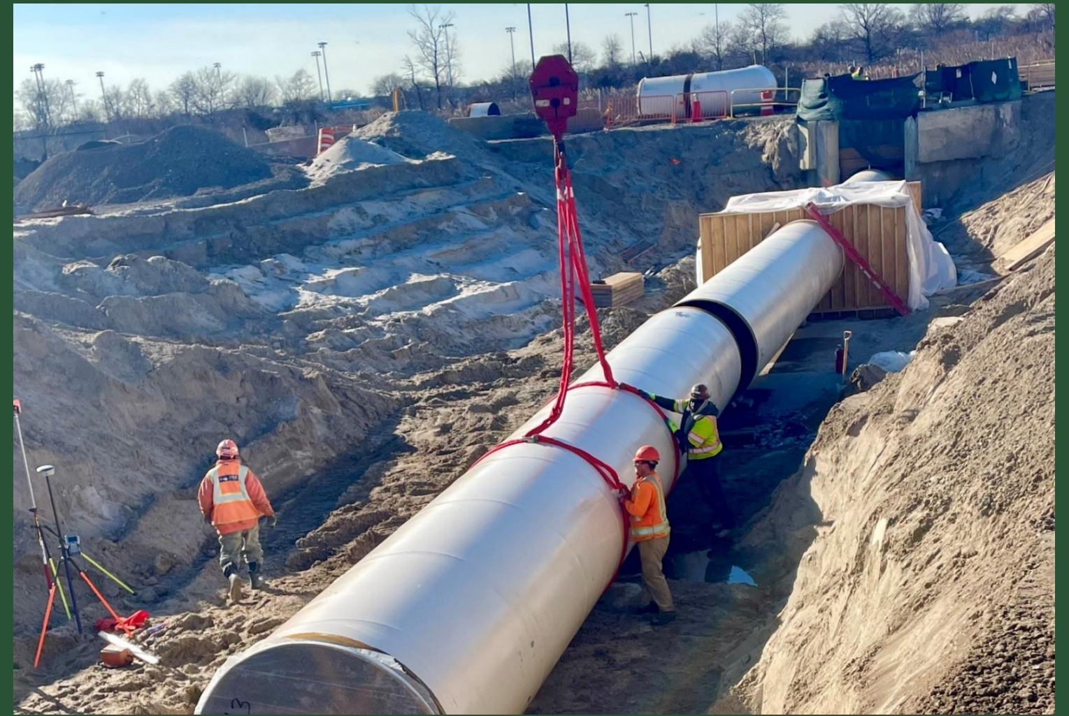
Pipe Connection to CC1 (January 2024)
