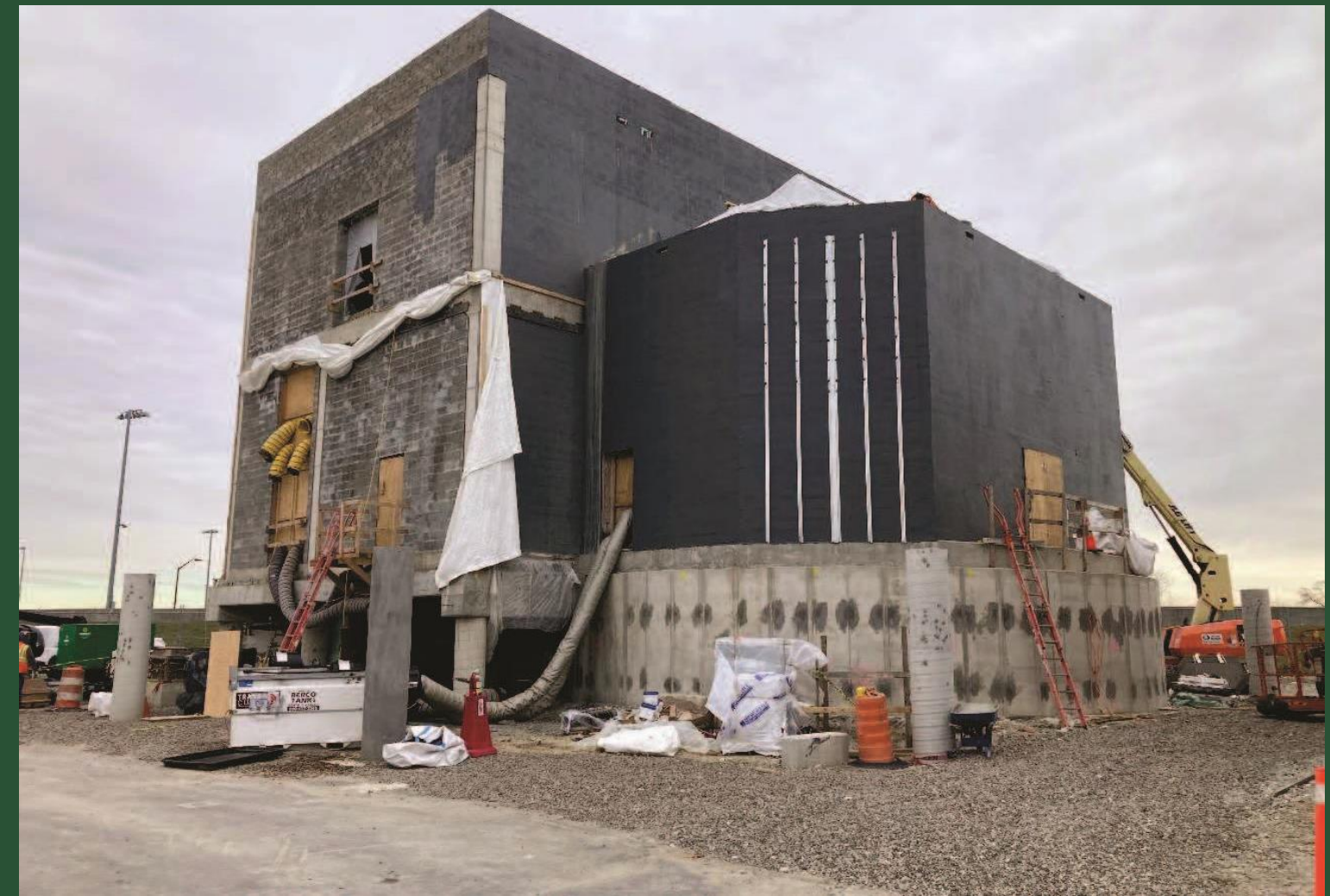
Pump Station Progress (January 2024)
