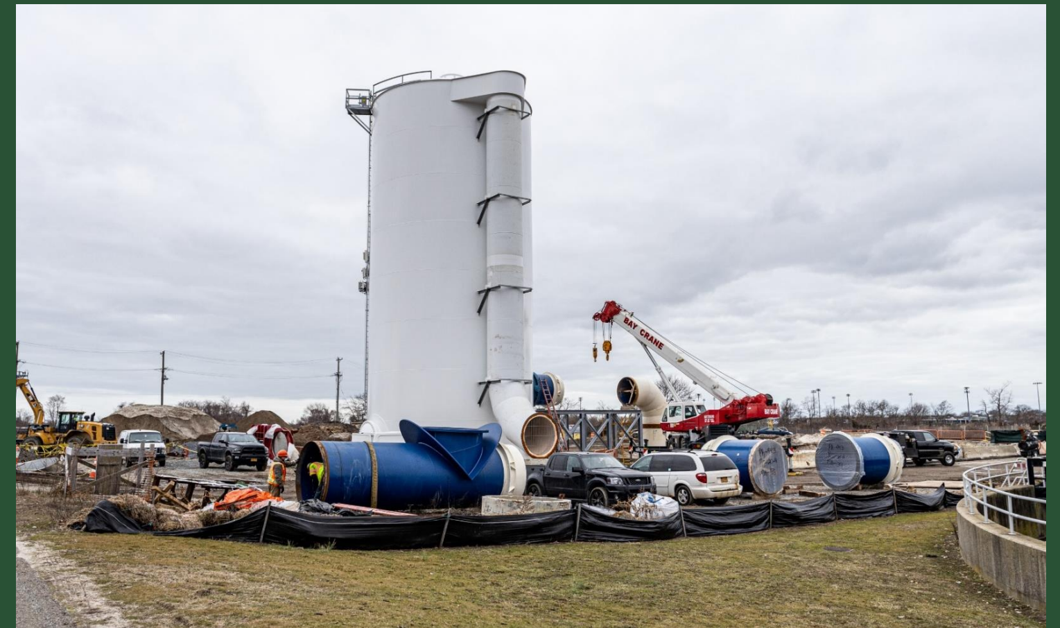
Receiving Tank Structure Progress (January 2024)
