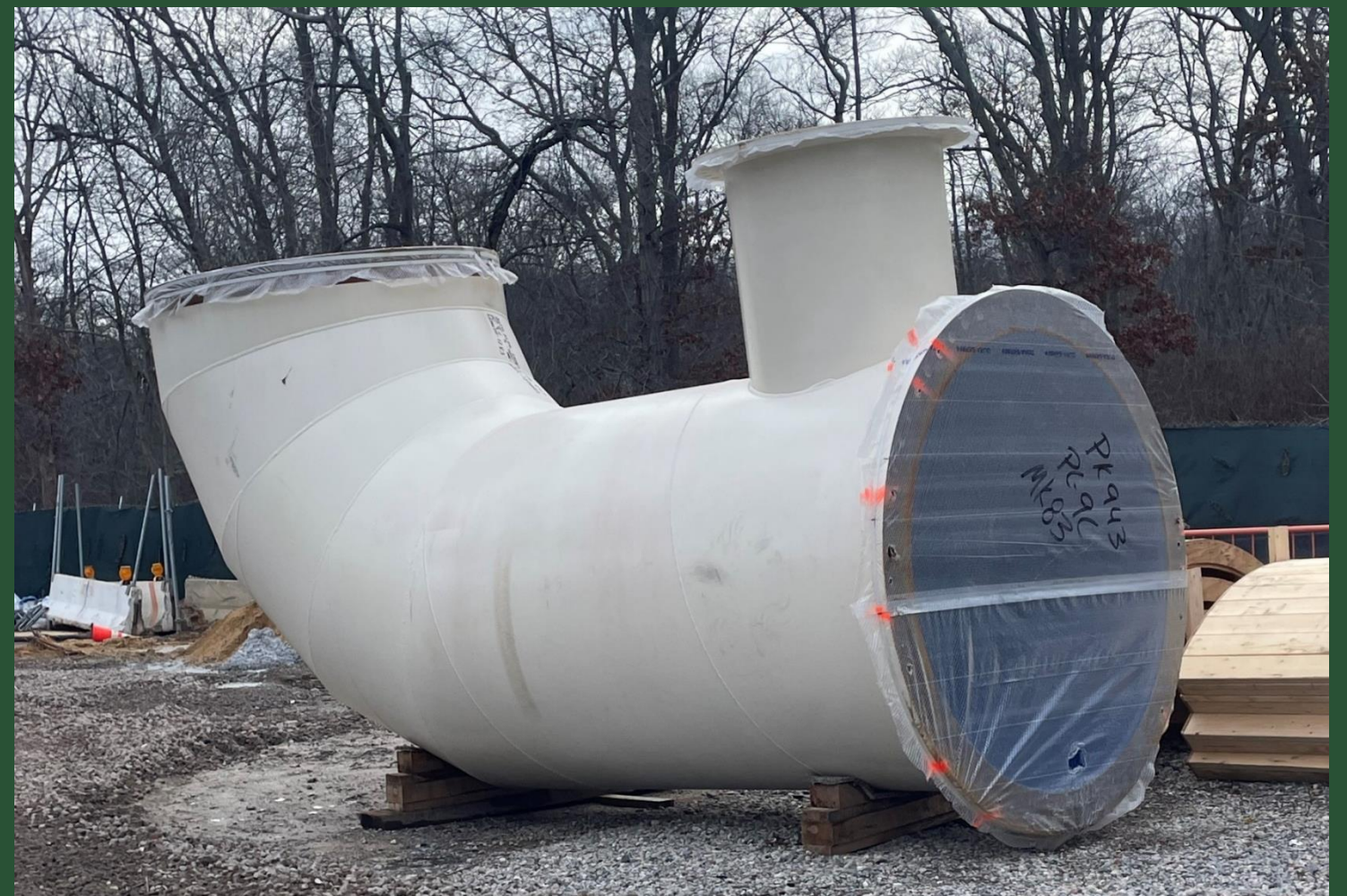
CC6 Riser Pipe (December 2023)
