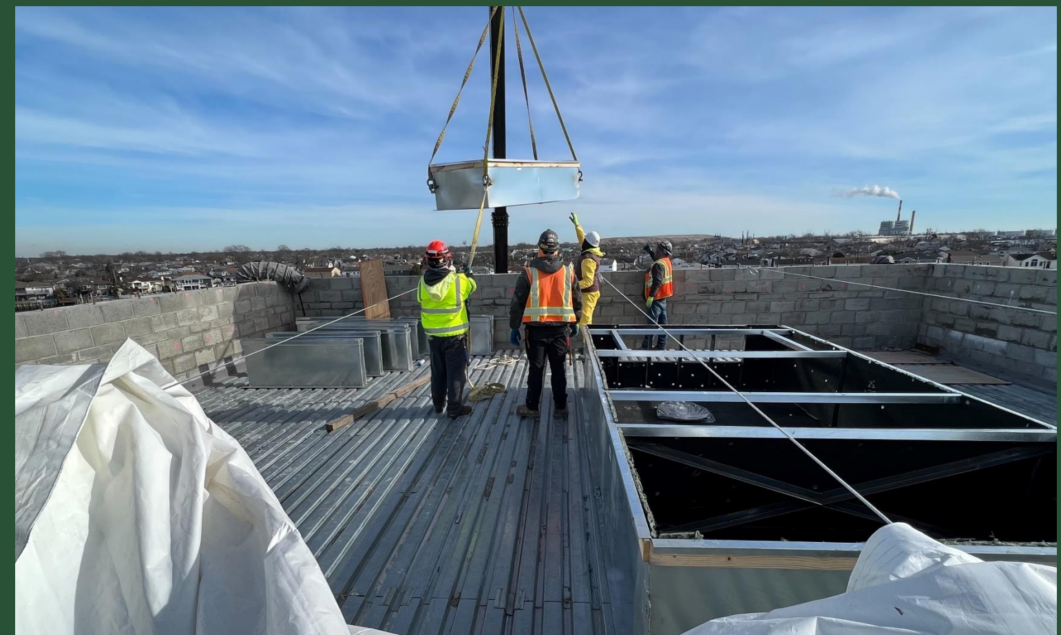
Roof Construction (December 2023)
