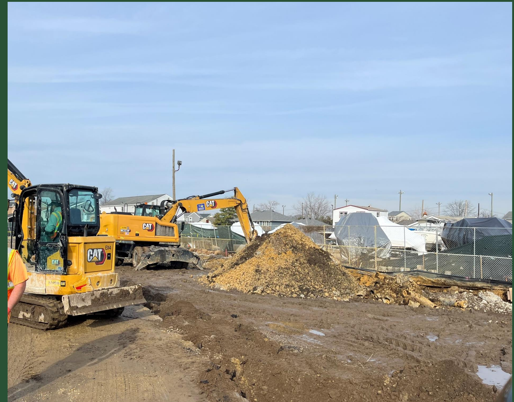
Grading at BP2 (January 2023)
