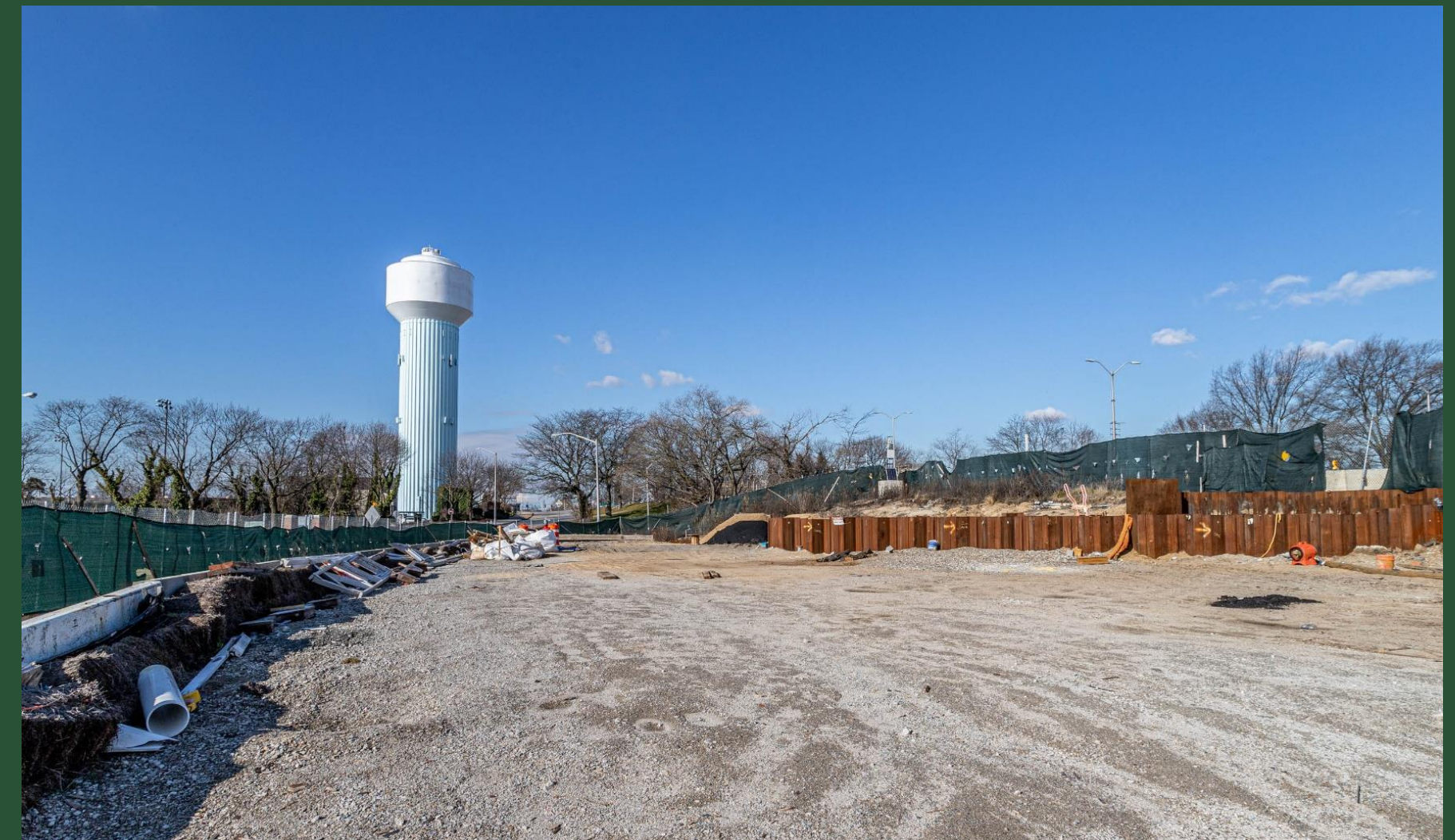
Construction Site at BP9 (January 2023)
