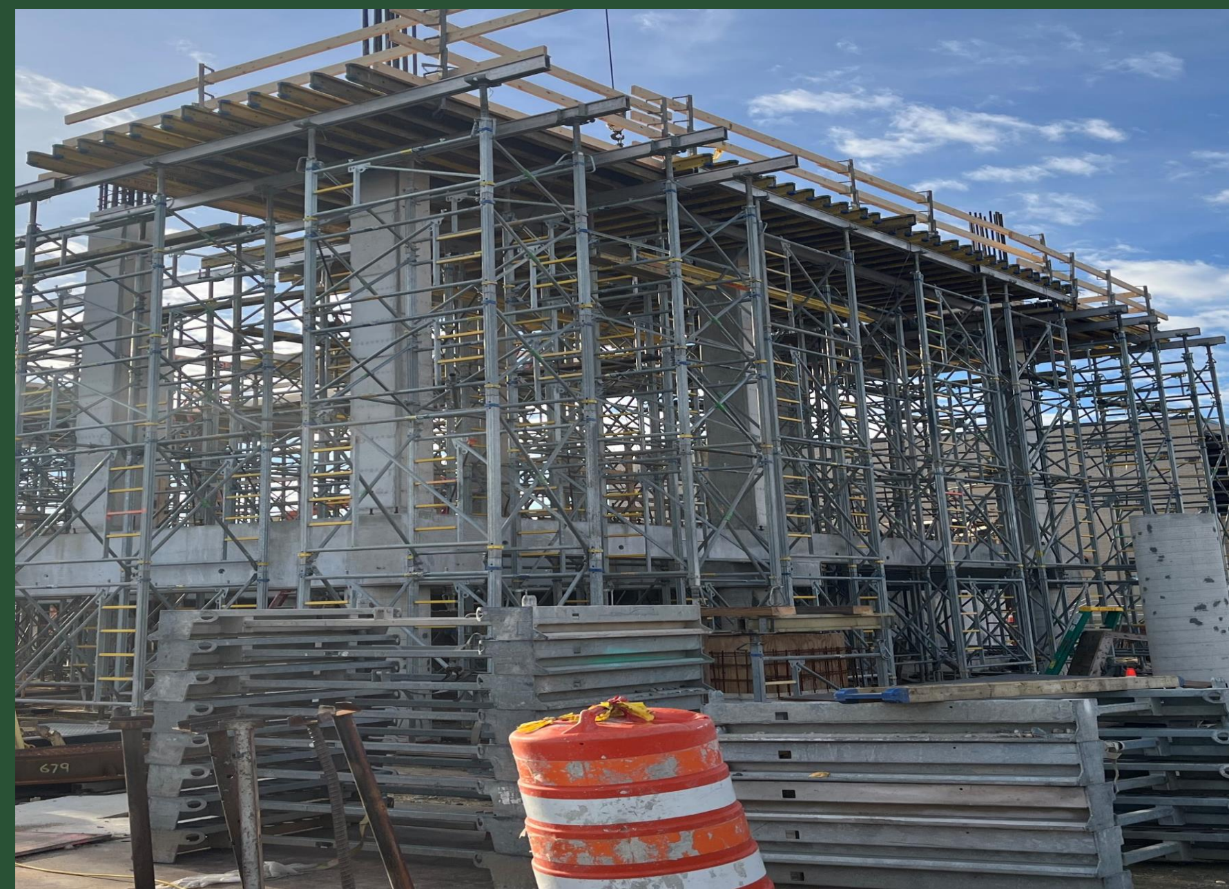
Pump Station Construction Near BP1 (February 2023)
