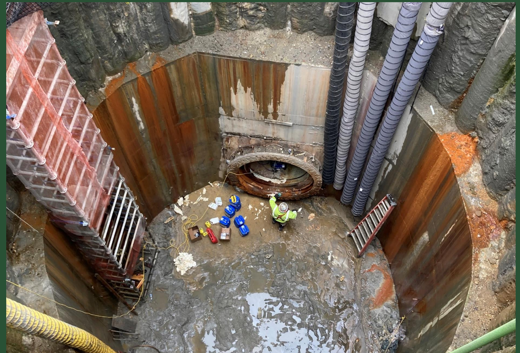
Post-Microtunneling Activities at CC2 (March 2023)
