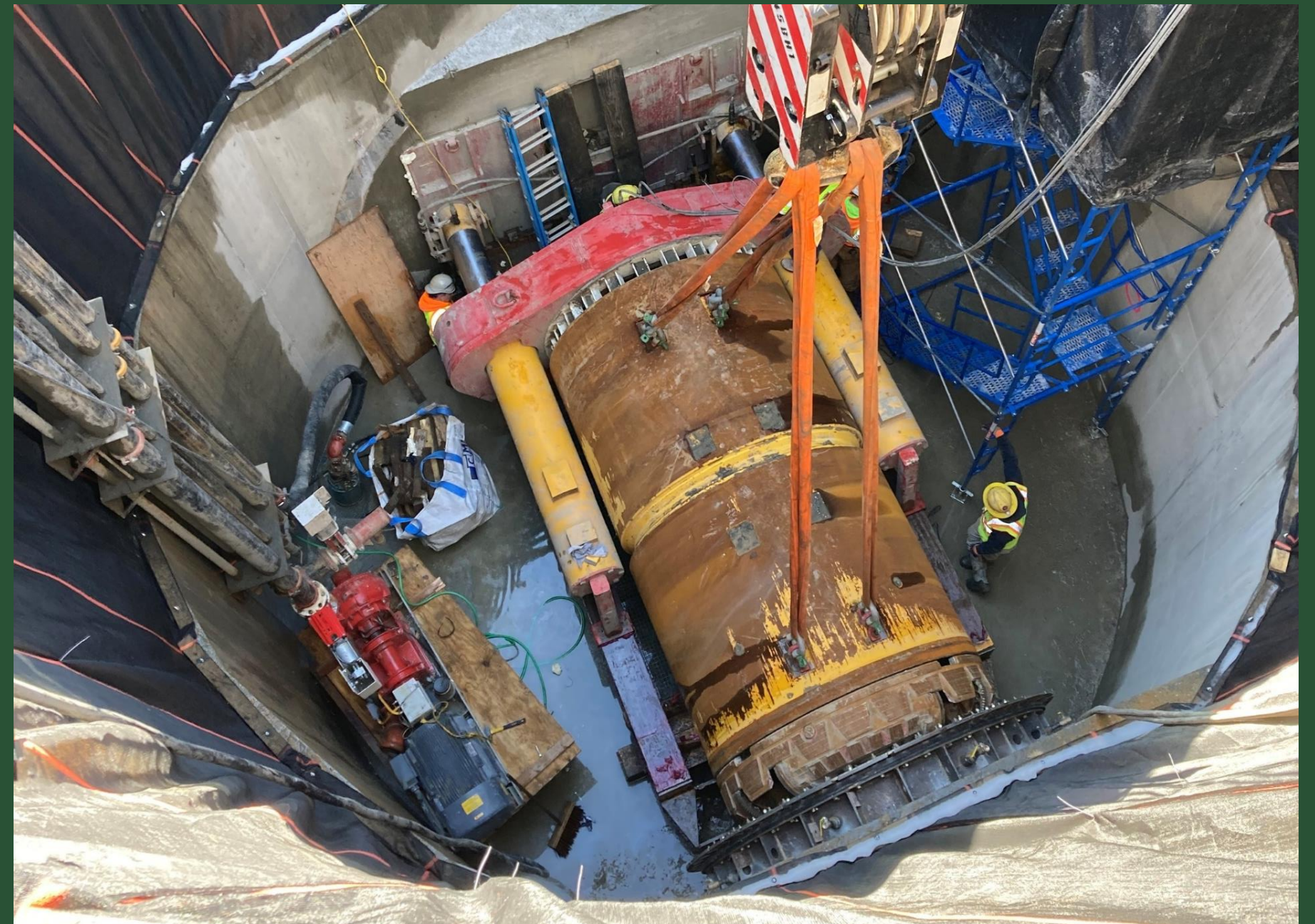
Preparation for Microtunneling from CC5 to CC6 (March 2023)
