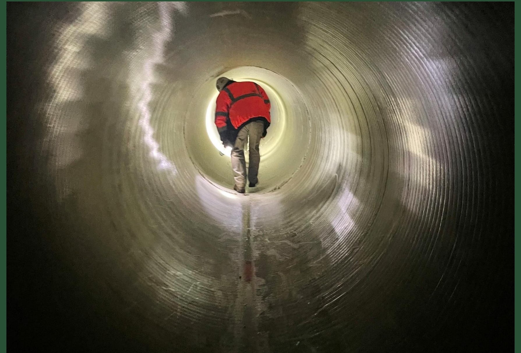
Inside the Conveyance Pipe near Pit I (February 2023)
