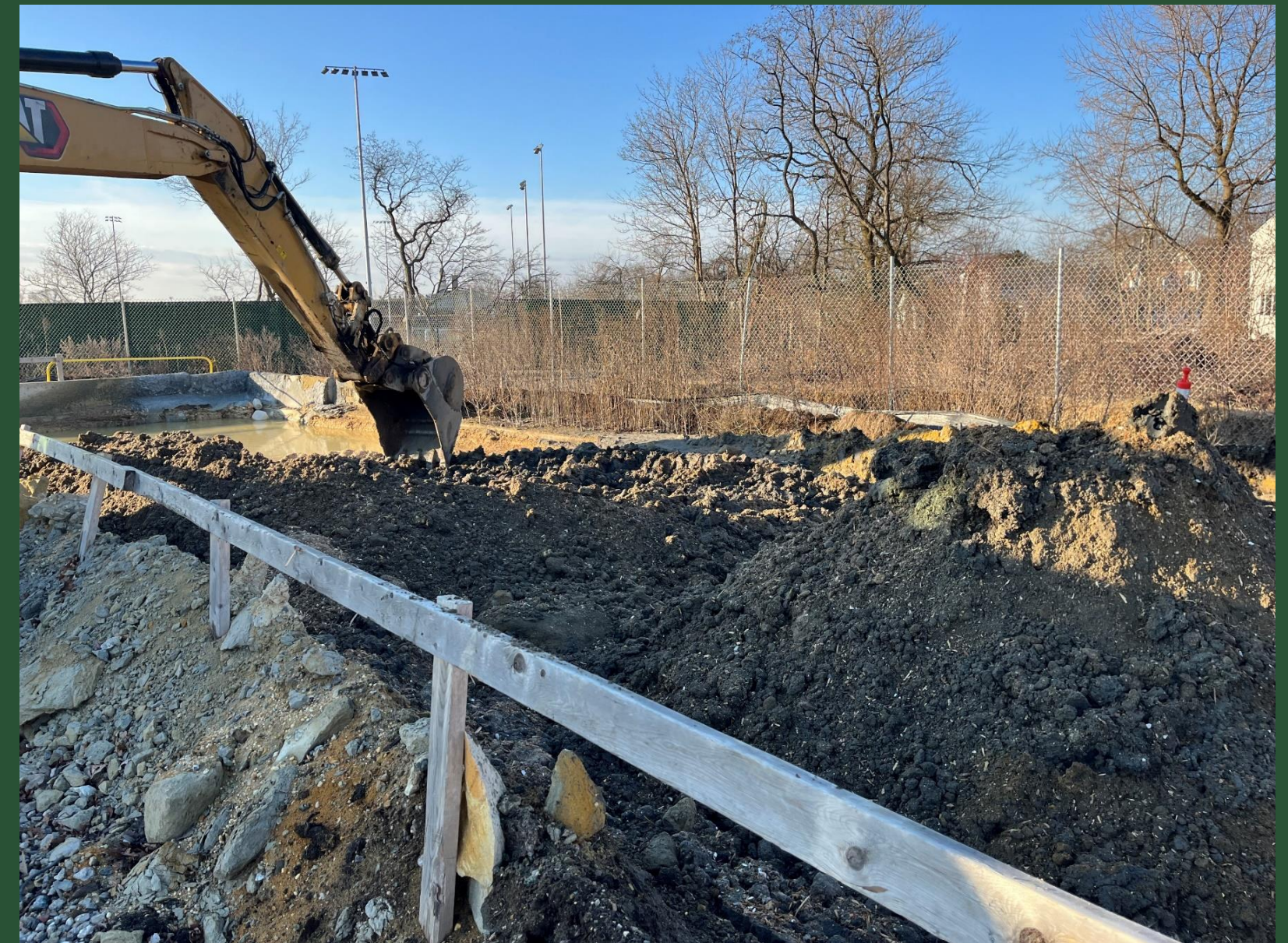
BP7 Spoils Removal (February 2023)
