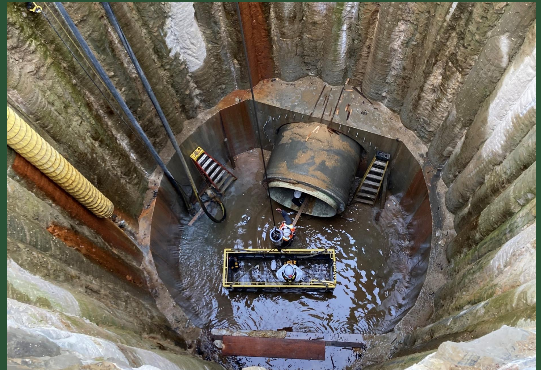
Seal Removal at CC3 ( February 2023 )
