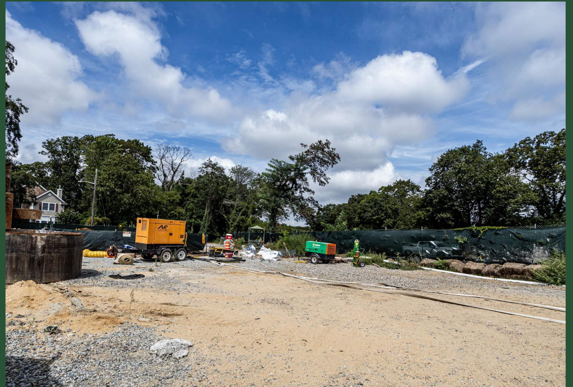
Grouting Activities at CC5 (August 2023)
