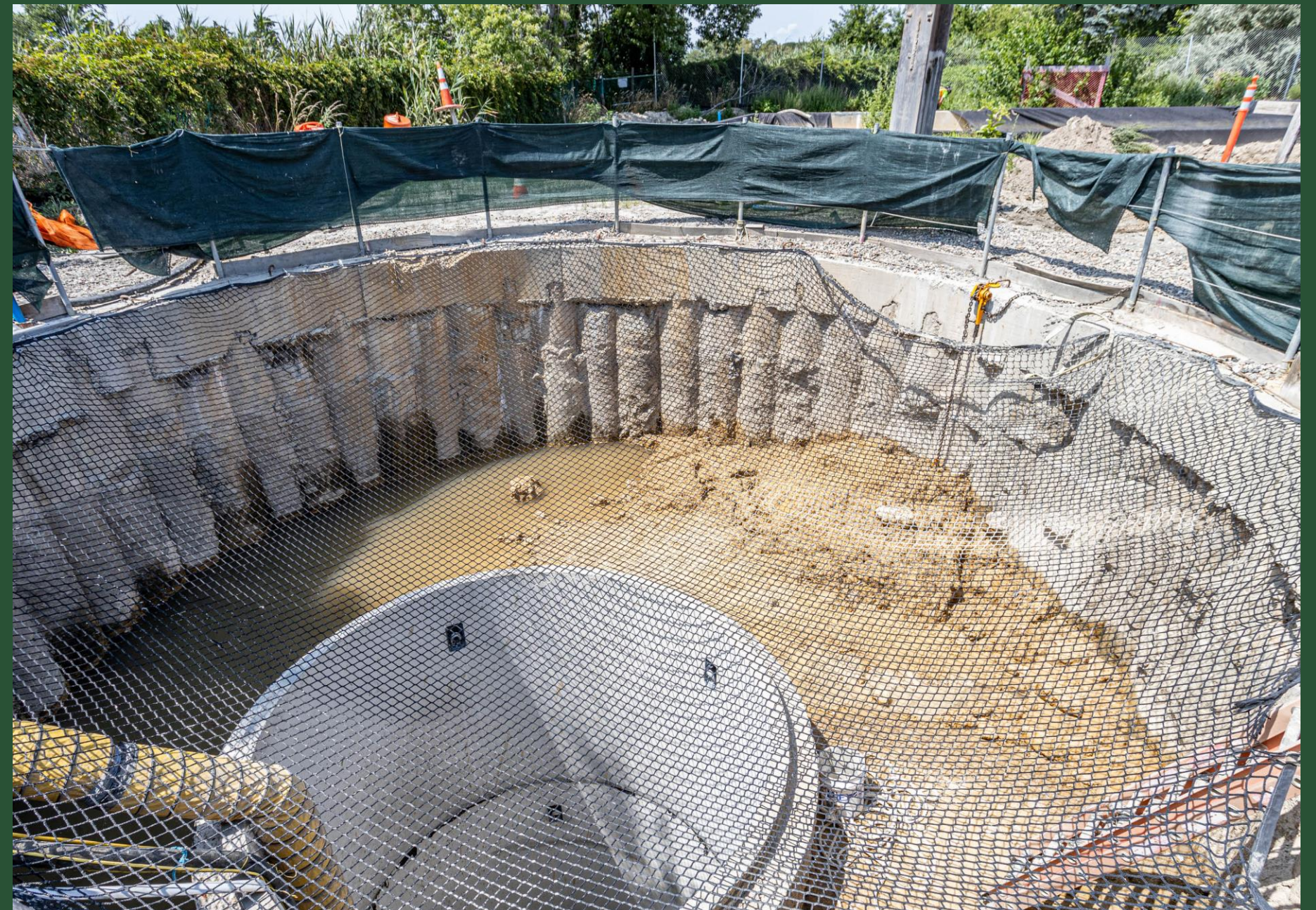
Backfilling at CC2 (July 2023)
