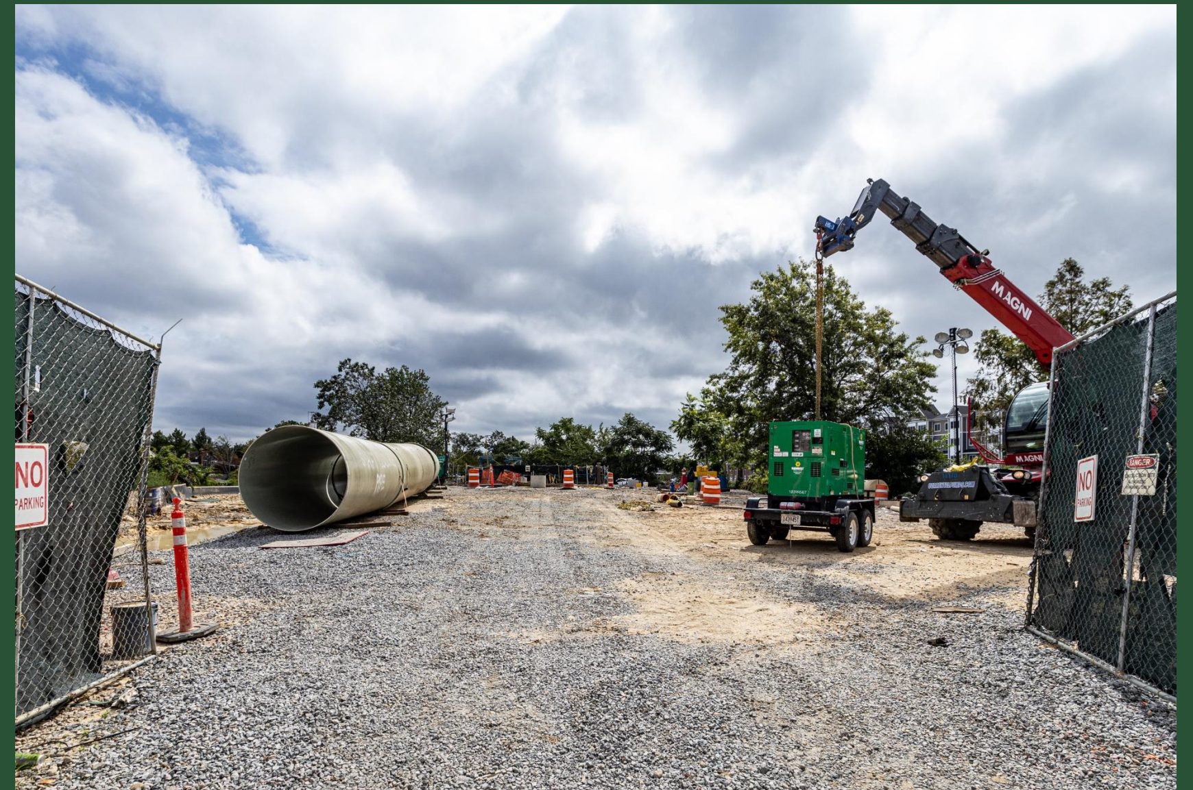
BP3 Restoration Activities (July 2023)
