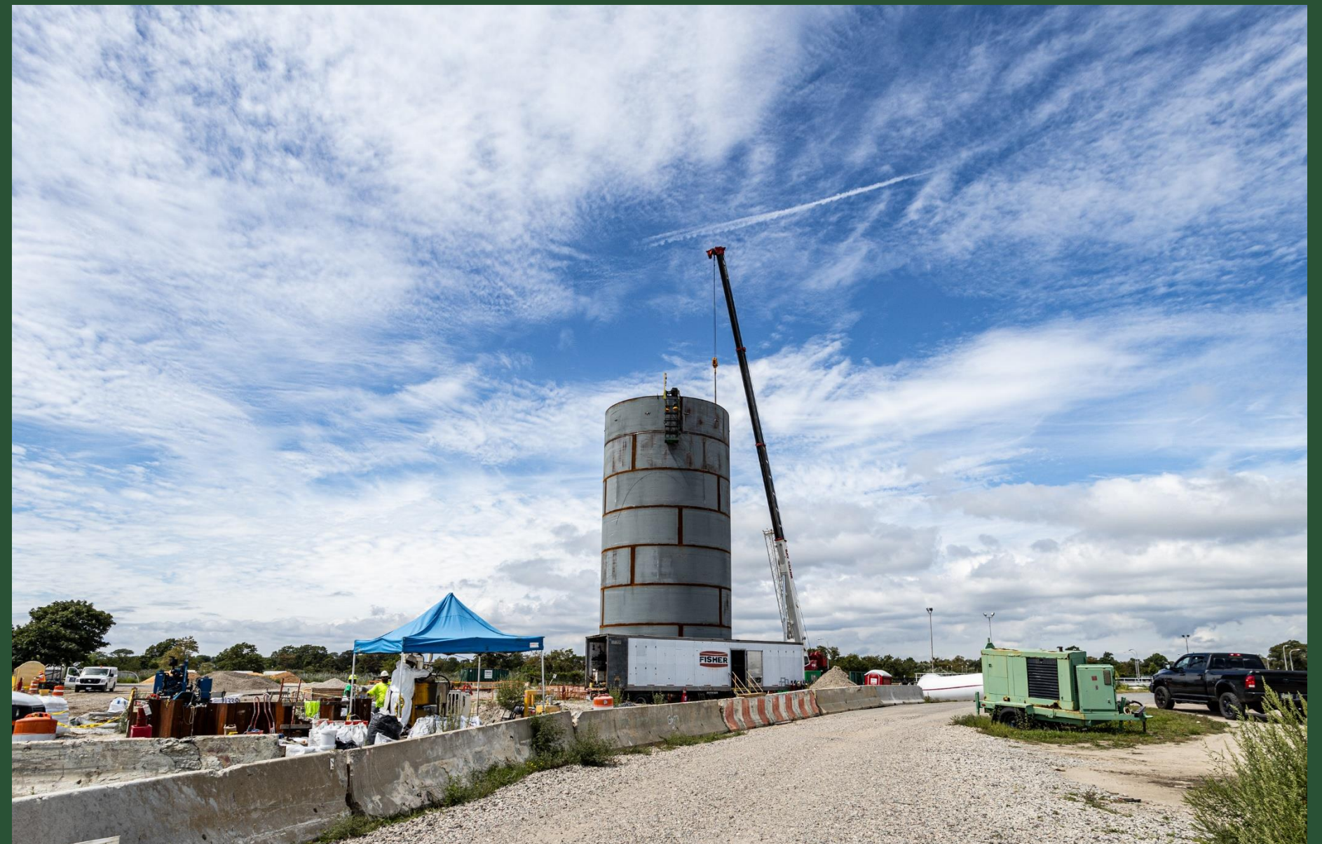
Receiving Tank Structure near CC1 (August 2023)
