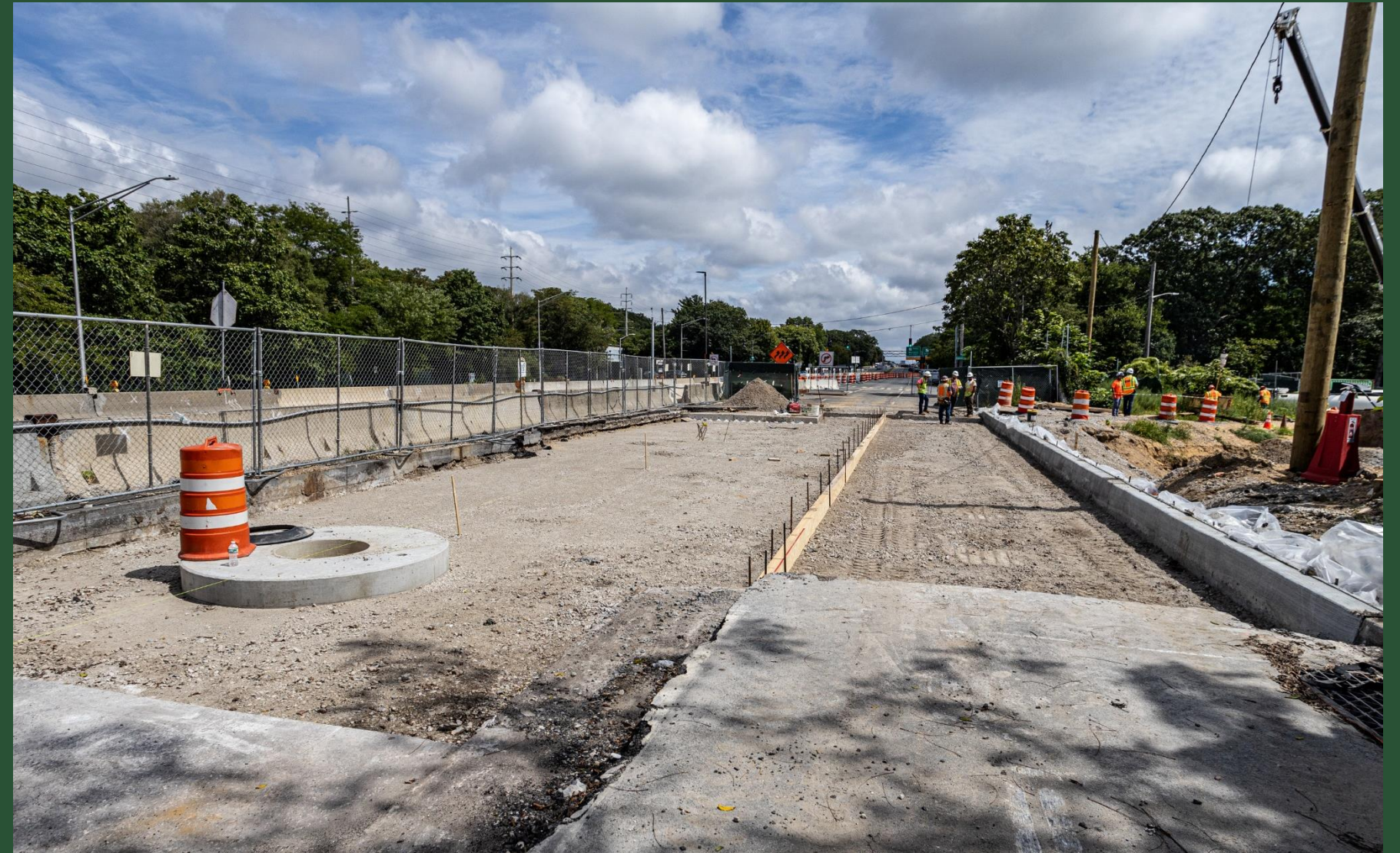
Construction at Pit W (September 2023)
