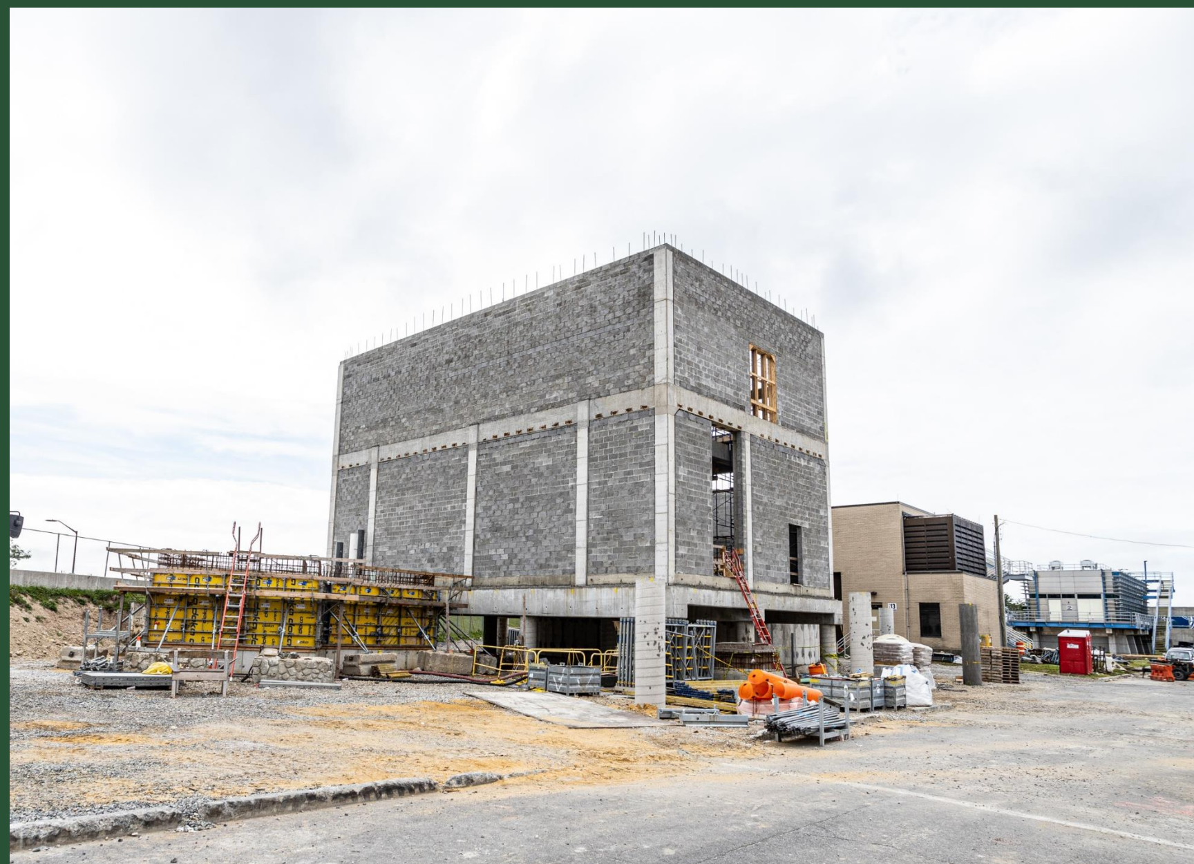
Pump Station Construction Near BP1 (July 2023)
