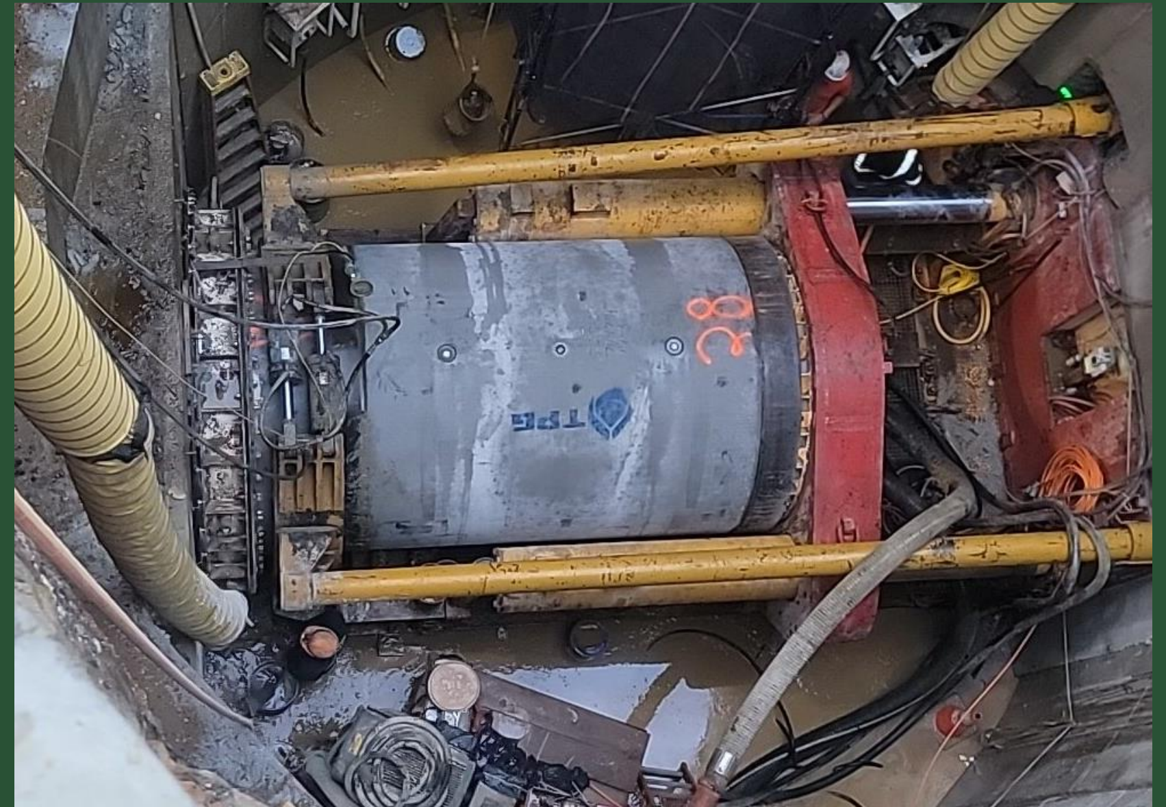
Microtunneling at BP8 (September 2023)
