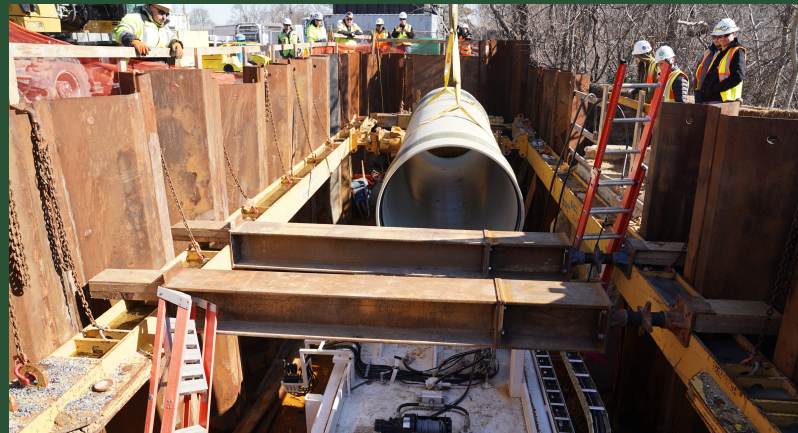
Start of Sliplining at Pit O (March 2022)
