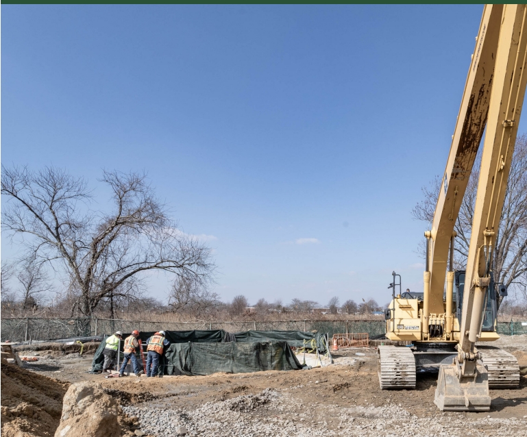
Shaft Excavation at CC2 (March 2022)
