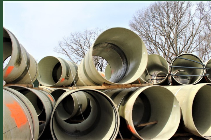
Pipe laydown area at Pit P (March 2022)
