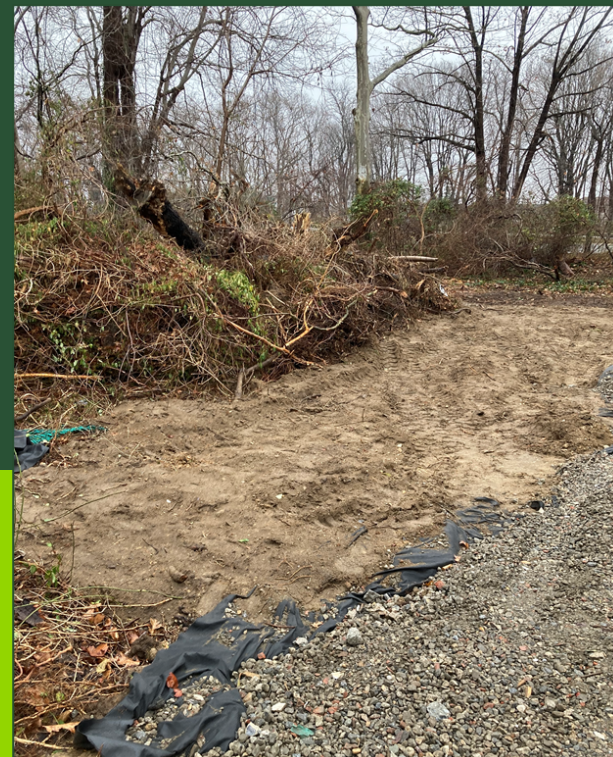
Clearing and Grubbing at CC4 (January 2022)
