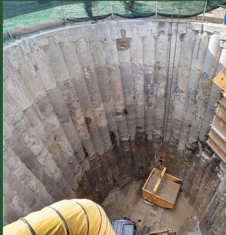
Shaft Excavation at CC1 (March 2022)
