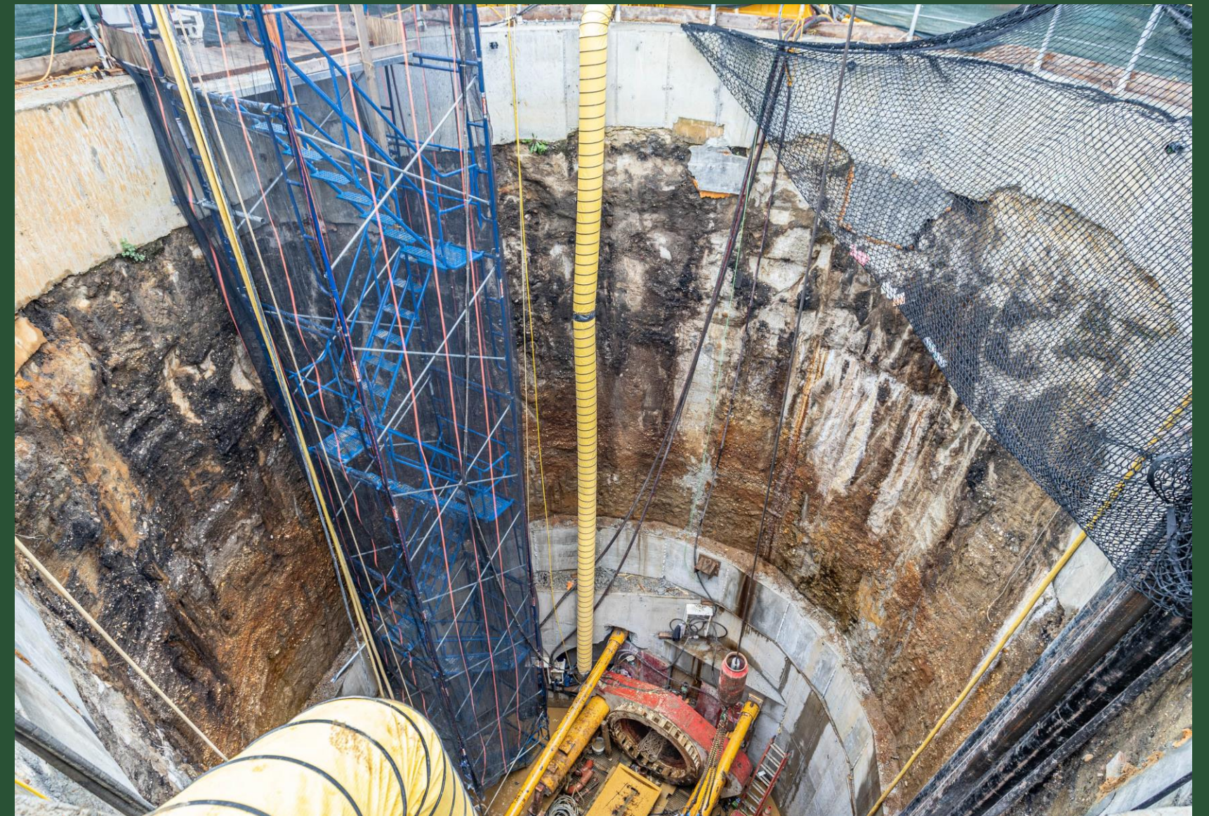
Microtunneling at BP8 (September 2023)
