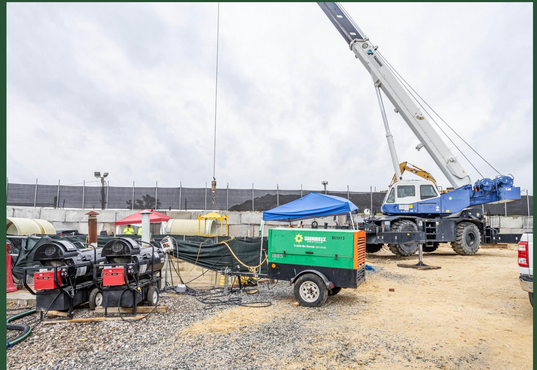
BP3 Restoration Activities (September 2023)
