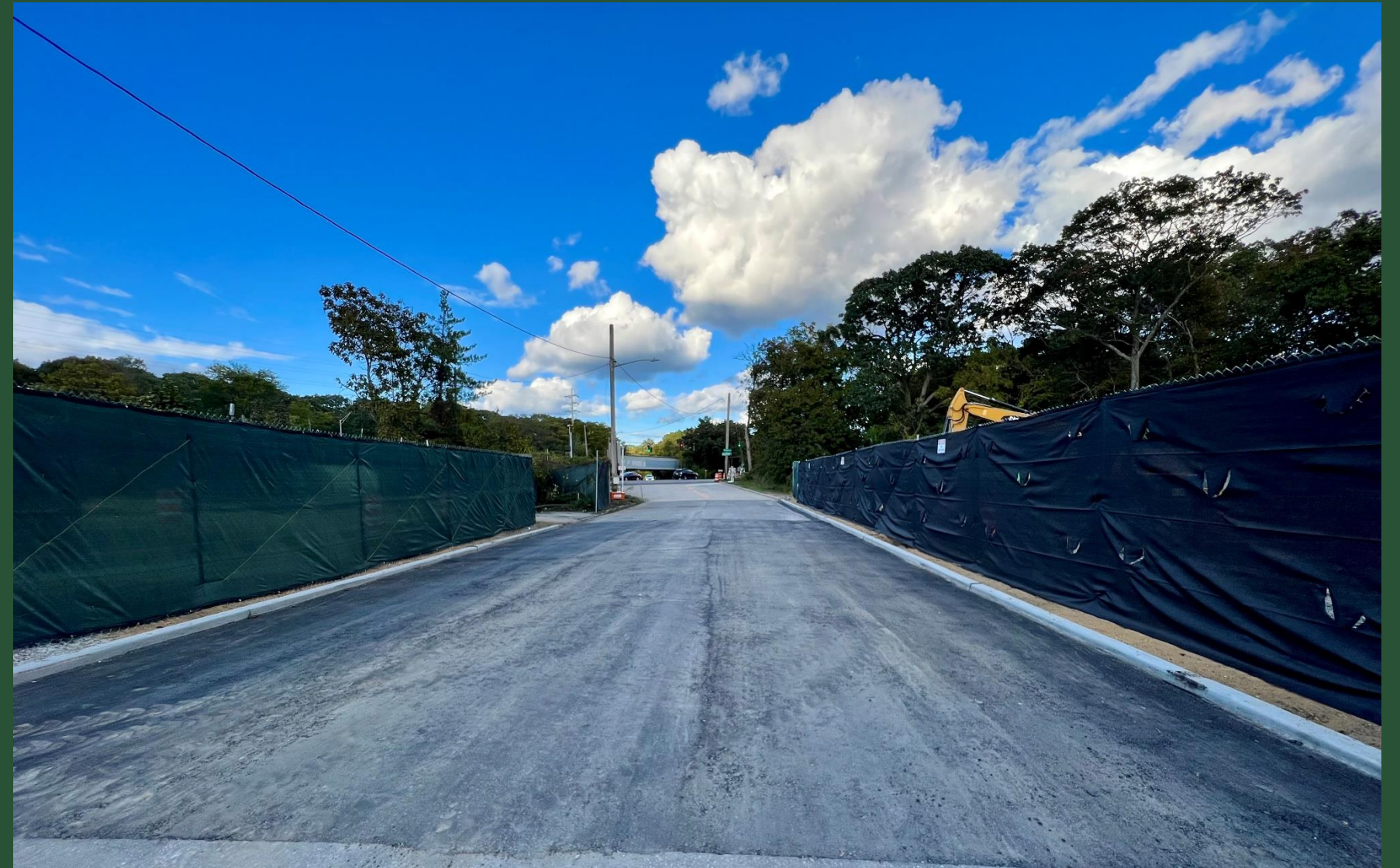
Lakeview Road Opening at CC6 and Pit W (October 2023)
