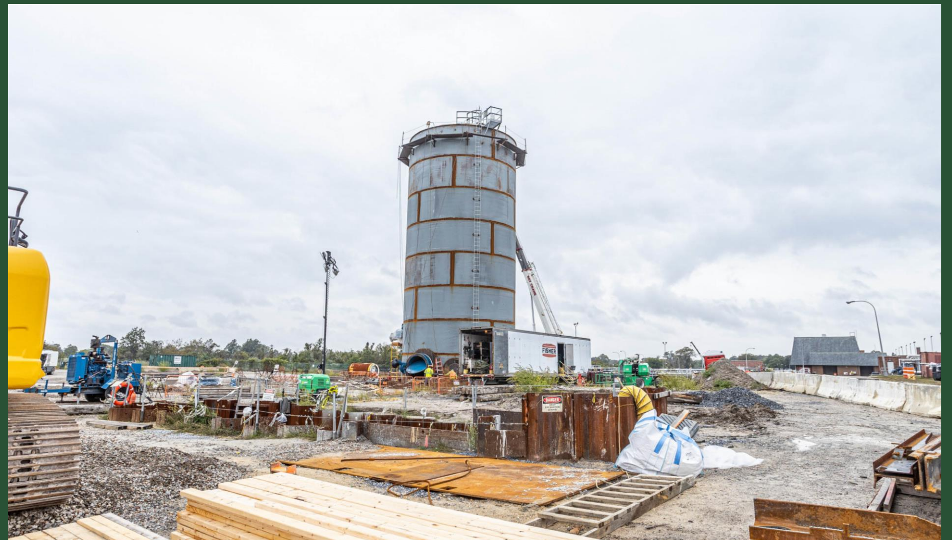
Receiving Tank Structure near CC1 (September 2023)
