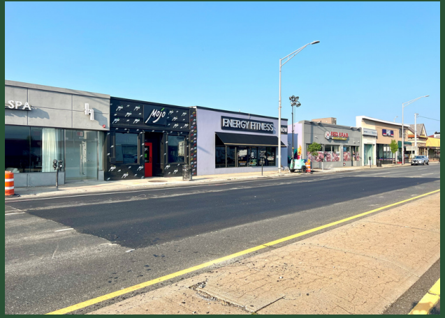
Roadway Restoration at Pit C (July 2023)
