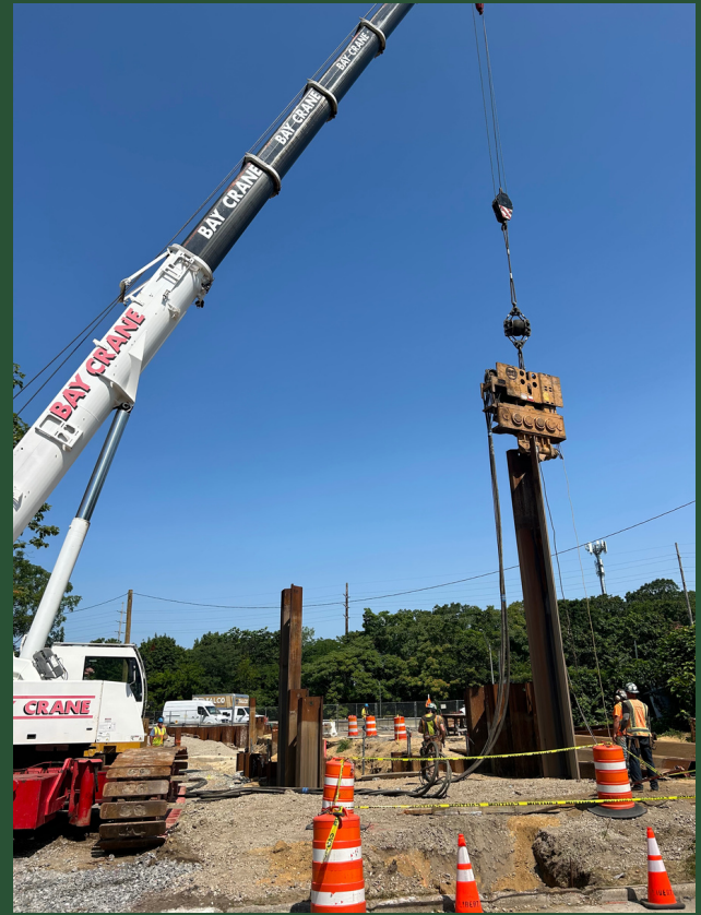
Sheet Pile Installation at Pit W (July 2023)
